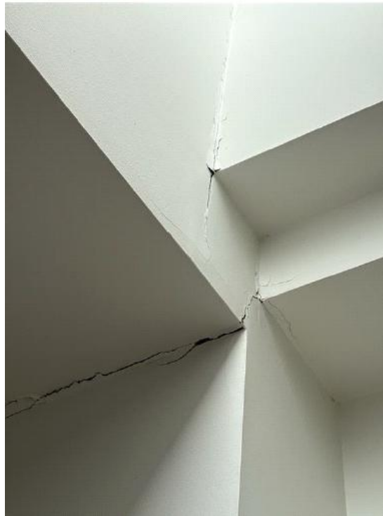
Close up of support beam seating
