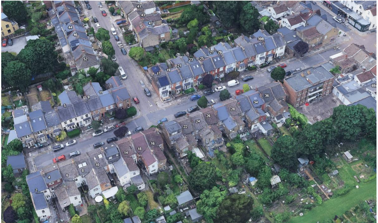
Image above from Google earth, shows Marlborough Road with a variety of different roof tiles and a number of rooflights and possibly solar panels to no 17.
