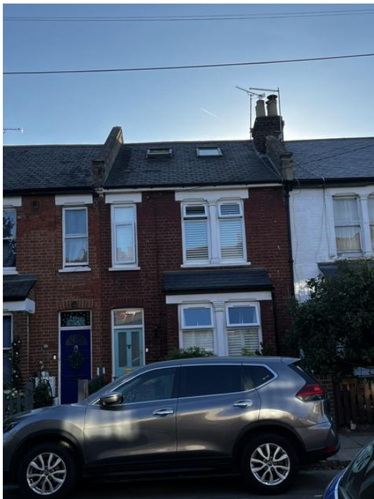
View of front façade of 27 Marlborough Road - there are already rooflights installed in the roof which were given planning permission (see Design and Access statement)
