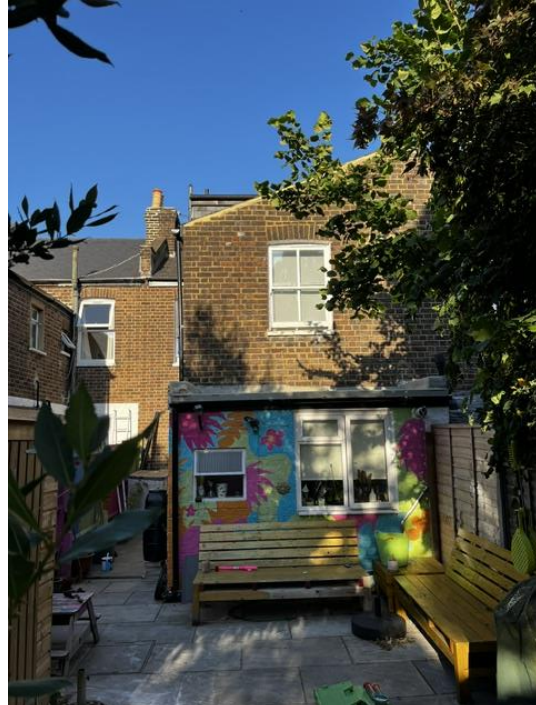
View of rear façade of 27 Marlborough Road
