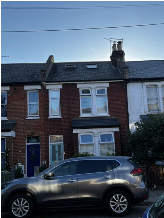
View of front façade of 27 Marlborough Road
