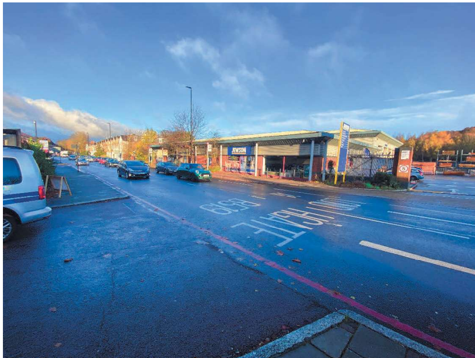
Photograph 06: View of the road outside the entrance to the Site.
