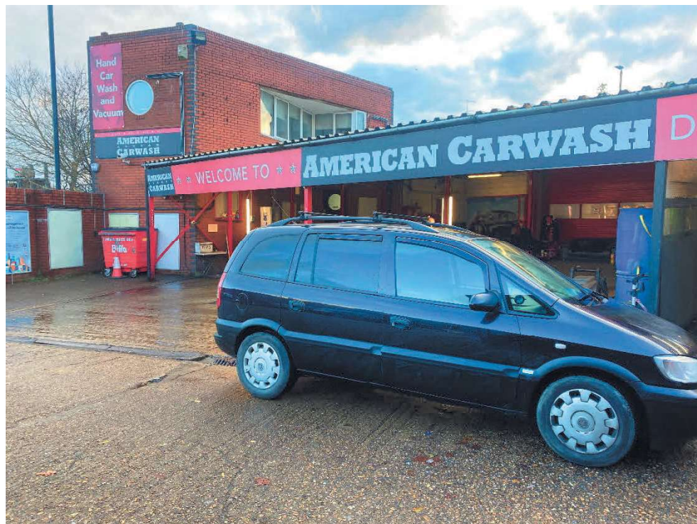
Photograph 02: View of the car wash area looking south-east.
