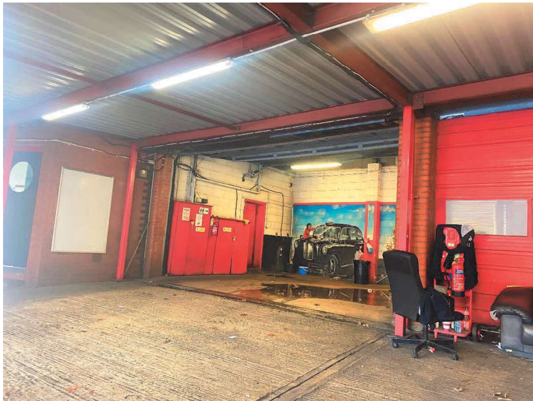
Photograph 03: View of inside the car wash area.
