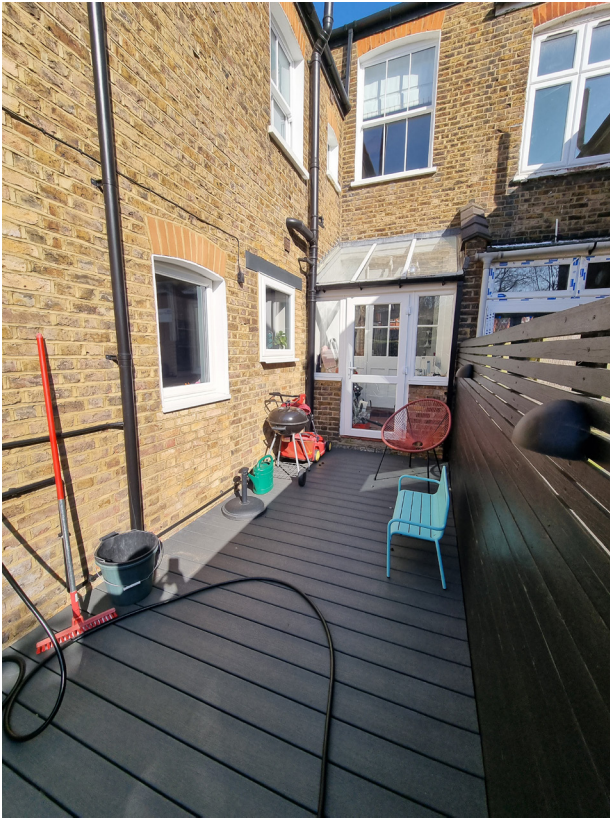
[Fig. 05] Rear facade view to 17 Barratt Avenue
