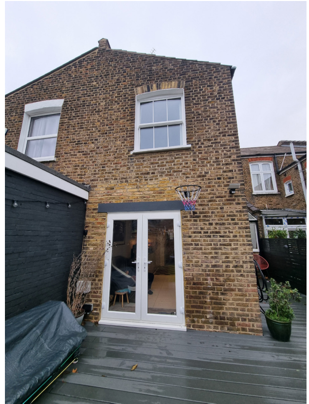
[Fig. 06] Rear facade view to 17 Barratt Avenue and relationship at boundary with No. 19.
