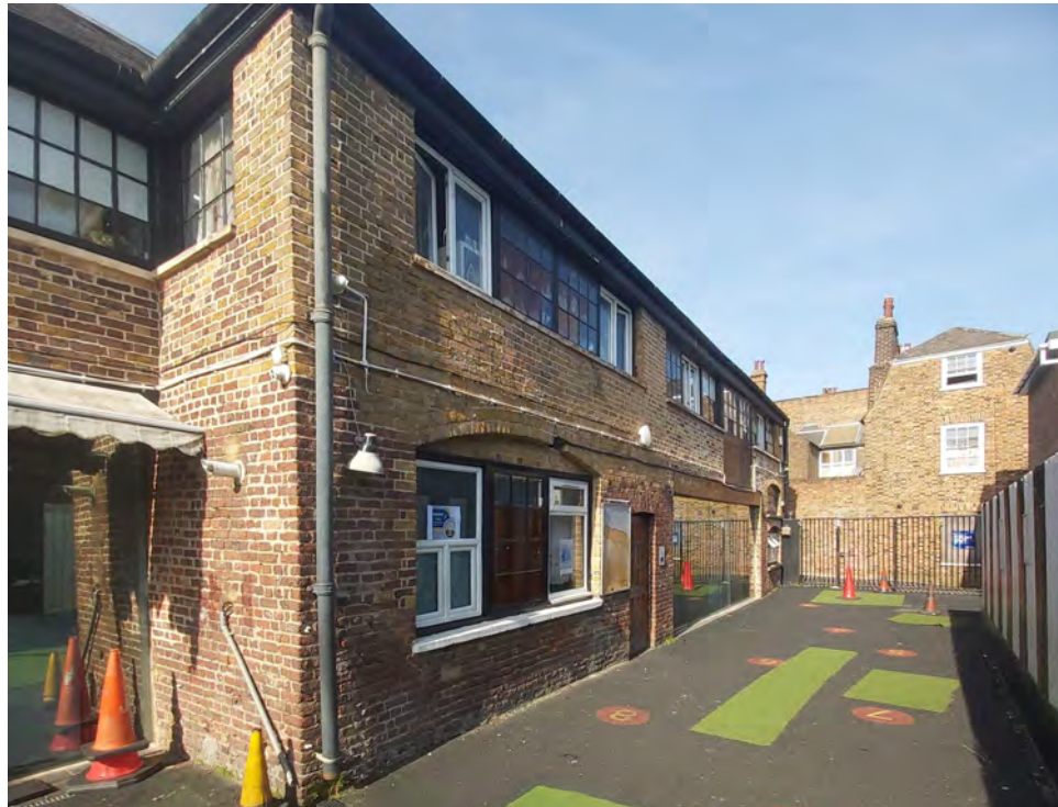
Locally Listed Building, looking North.
