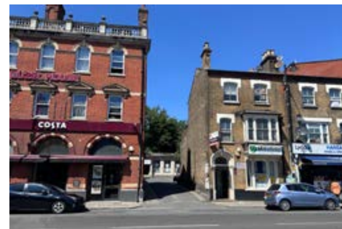
Figure 3.8 Access to 551B High Road, south of the Site Source: Author [Dated: 25.08.2024]
