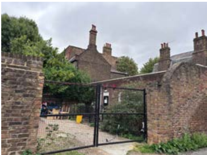
Figure 6.11 View of rear gardens behind No 581, now lost as part of the later development of Ashling House, Kenmare Drive. Source: Author [Dated: 25.07.2025]
