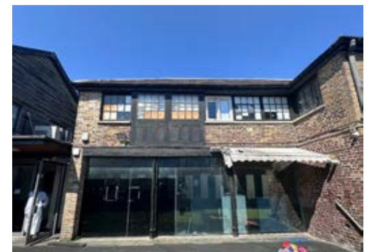
Figure 5.7 Southern part of the eastern elevation of the 19th Century part of the Barn, showing UPVC window on the first floor. Source: Author [Dated: 25.07.2025]
