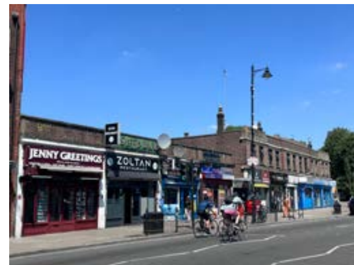
Figure 6.5 Nos 559-565 High Road, part of a single storey range constructed in 1950, creating an unlikely gap in the street frontage. Author [Dated: 25.07.2025]
