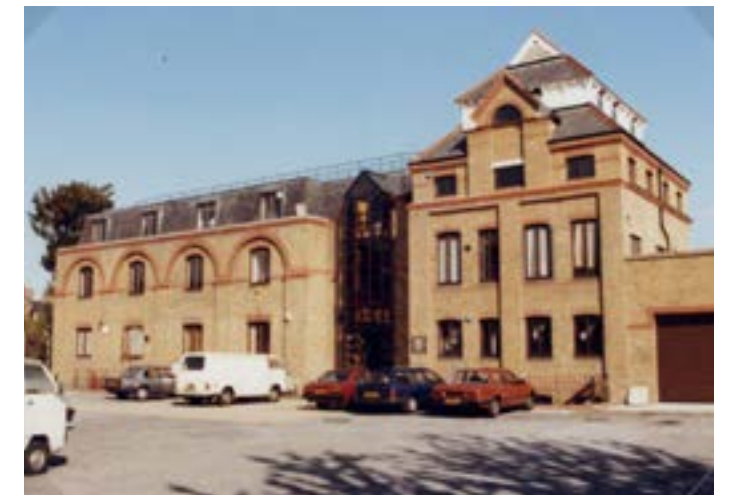
Figure 6.18 1981 Comparative view of the former brewery at 551a High Road. After remaining vacant the building was subsequently damaged by fire in 1981 (top). Planning permission for its conversion to light industrial use and extension was granted in 1981 (bottom). Source: With permission from London Metropolitan Archives (not to be reproduced)
