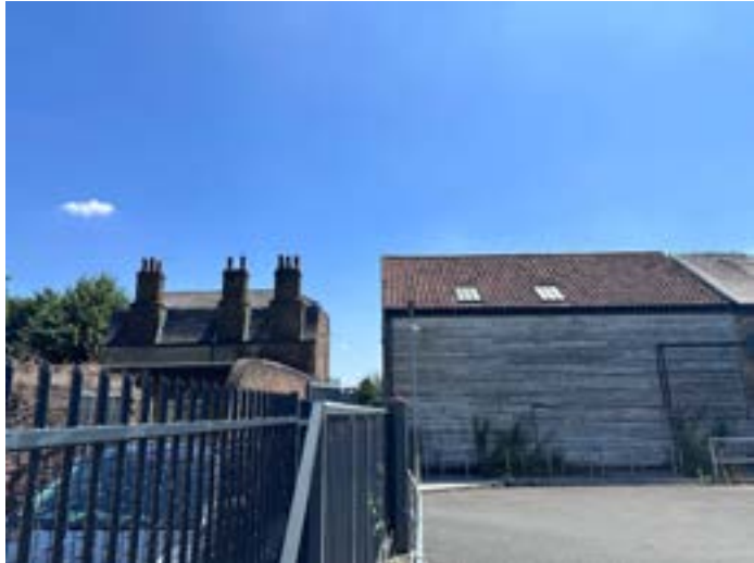
Figure 6.12 Rear elevation of the Barn with the rear of No 581 to its left, taking from the parking of Charlton Medical Centre. Source: Author [Dated: 25.07.2025]
