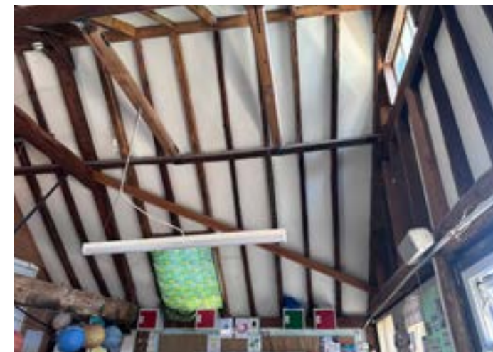
Figure 5.10 Internal view of first floor room within the 18th Century Barn part of the Barn, used as classroom. Source: Author [Dated: 25.07.2025]
