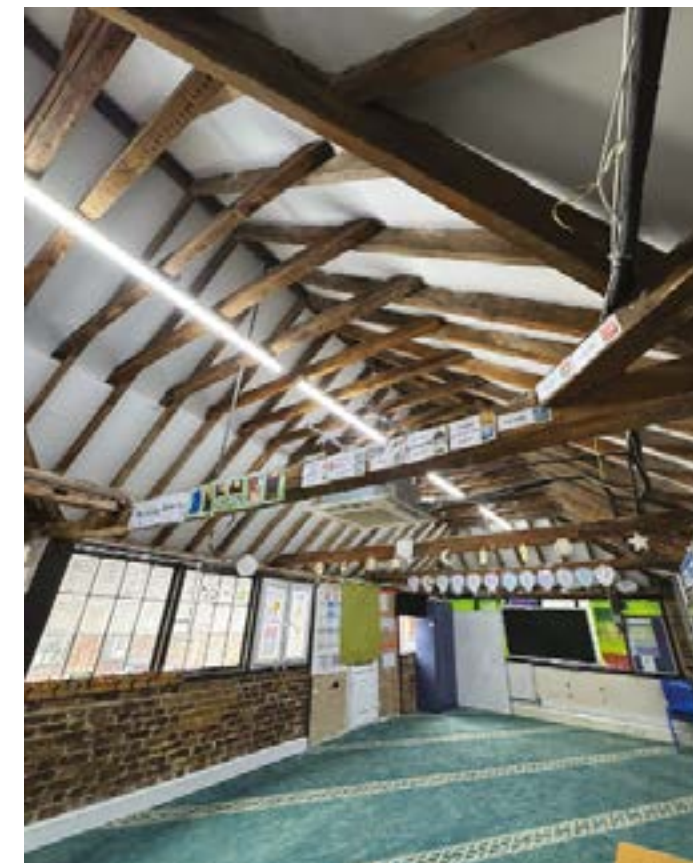
Figure 5.12 Internal view of the classroom within 19th Century extension. Source: Author [Dated: 25.07.2025]
