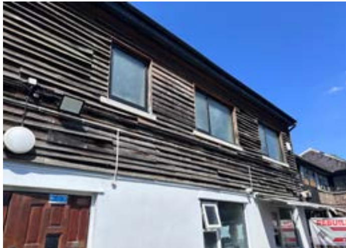
Figure 5.13 Eastern elevation of the 2004 office extension, showing later UPVC windows and slipping timber cladding. Source: Author [Dated: 25.07.2025]
