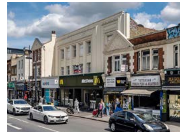
Figure 3.5 Terraces to the south of High Road, opposite Bruce Grove Station Source: Author, July 2025
