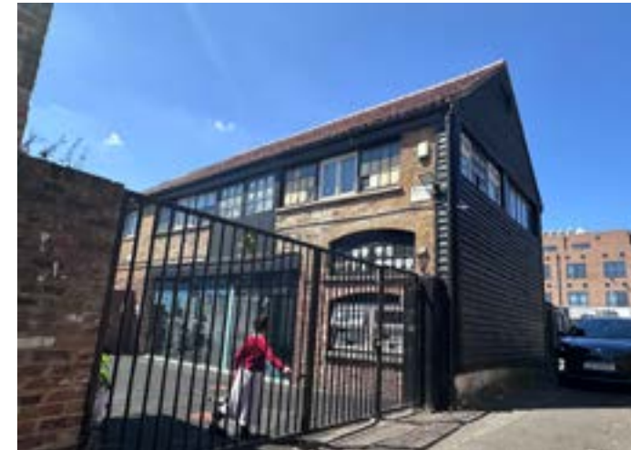
Figure 5.17 Western elevation of the Barn, seen from the drive way into the parking of the Medical Centre. Source: Author [Dated: 25.07.2025]
