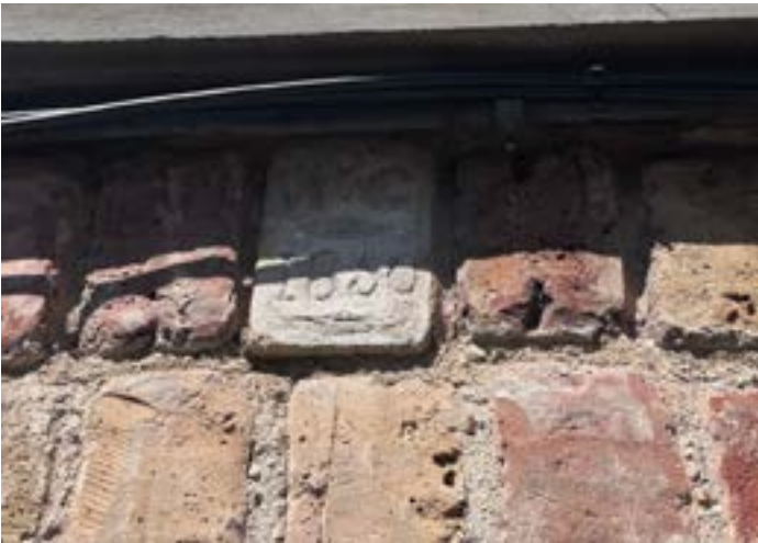
Figure 5.3 Date stone (1850) over the Northern part of the 18th Century Barn's eastern elevation, over the lower brick arch (see fig 3.10). Source: Author [Dated: 25.07.2025]
