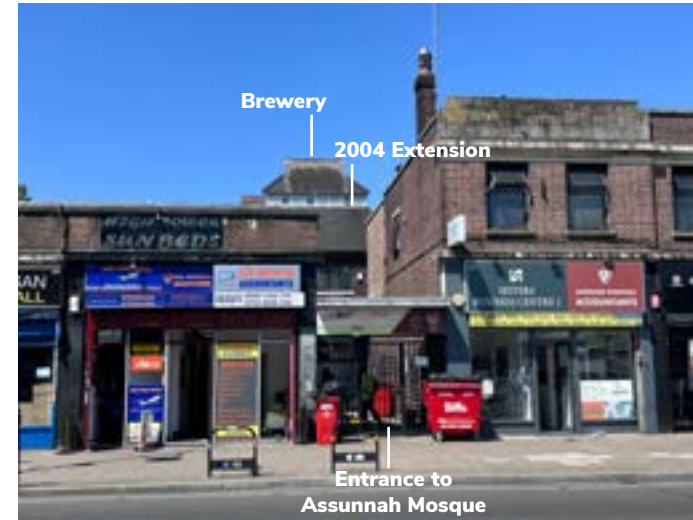
Figure 6.4 Entrance gates to Assunnah Mosque from High Road between Nos 565 and 567 High Road. Author [Dated: 25.07.2025]
