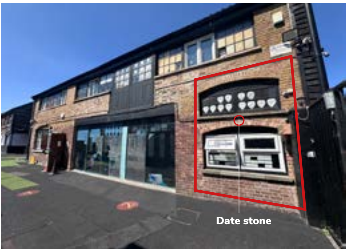
Figure 5.4 Northern part of the eastern elevation of the earlier 19th Century part of the Barn. The highlighted part in red would have contained a single storey range running perpendicular. The variation in brick colour and arch height shows that the elevation was rebuilt after the single storey range were demolished. Source: Author [Dated: 25.07.2025]
