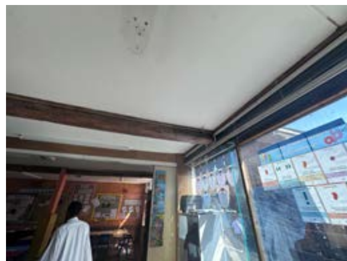
Figure 5.9 Internal view of the ground floor room within the 18th Century part of the Barn (south), used as a classroom. Source: Author [Dated: 25.07.2025]
