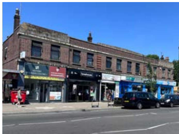
Figure 6.3 Nos 567-577 (Devonshire Terrace) High Road, a two storey terrace from 1930s containing retail premises on the ground floor and residential above. Source: Author [Dated: 25.07.2025]
