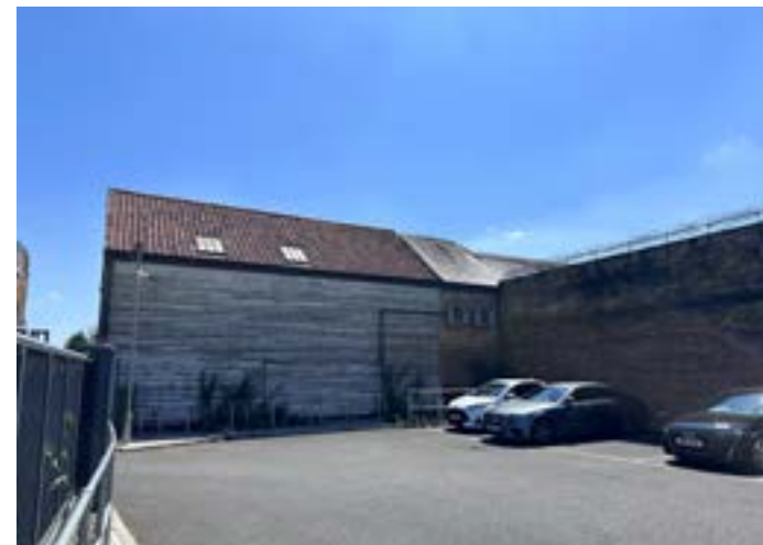
Figure 5.16 Western elevation of the Barn, seen from the parking of the Medical Centre. The timber clad and tiled roof part of the building is 18th Century; the brick and slate part is the 19th Century section. The wall forms the boundary to Morrison Yard. Source: Author [Dated: 25.07.2025]
