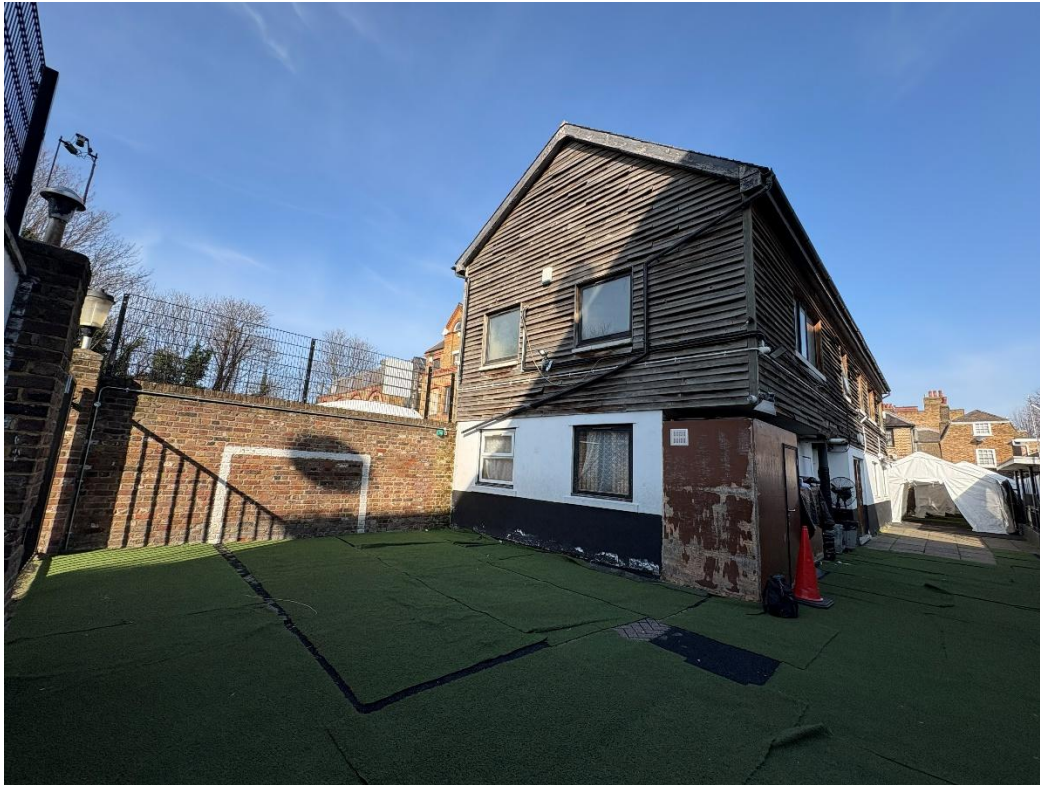
Photo 2: Front and southeast side of property (B1) viewed from southeast corner
