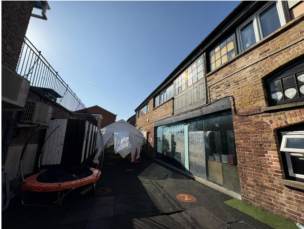
Photo 1: Front of property (B3) viewed from northeast
