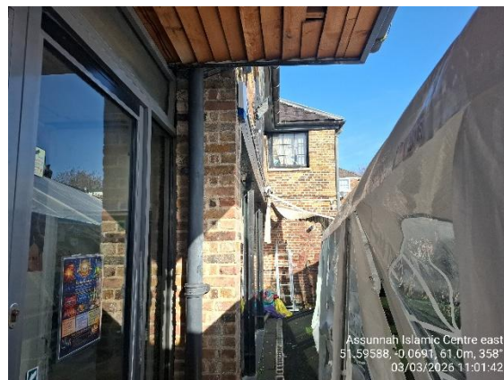
Image 5 – Building 2 (Aval Consulting Group, 2026)
