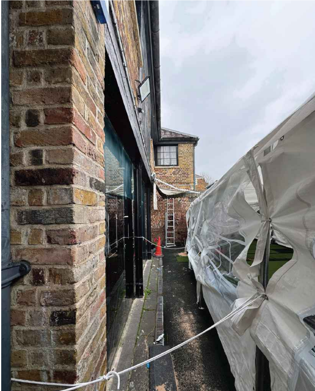
Photo 08 - Photo Looking North along East Elevation
