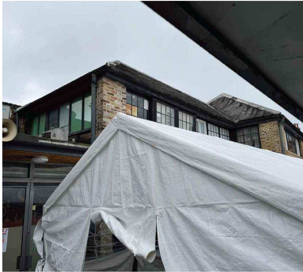
Photo 03 - View of South East Corner of the 19th Century Portions
