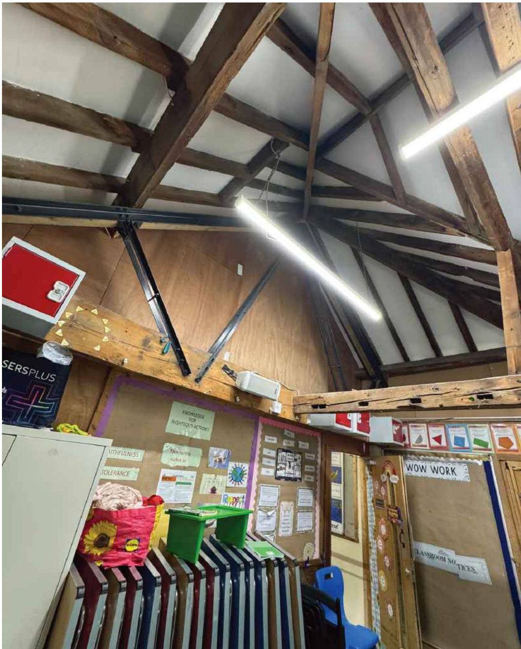
Photo 05 - Northern Portion of the Roof - Looking North
