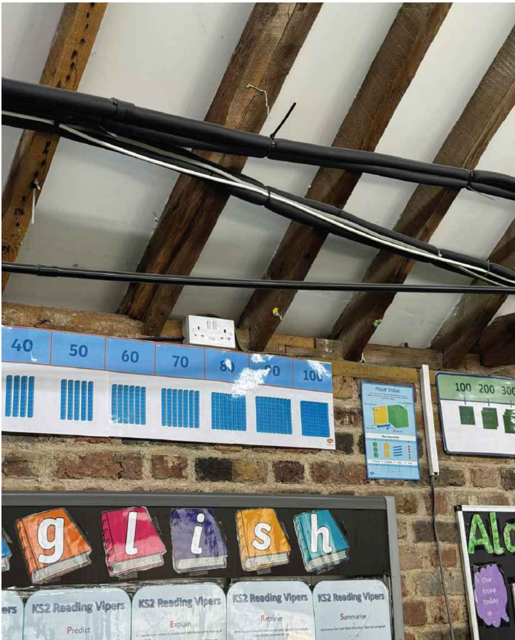
Photo 11 - First Floor - Timber Wall Plate
