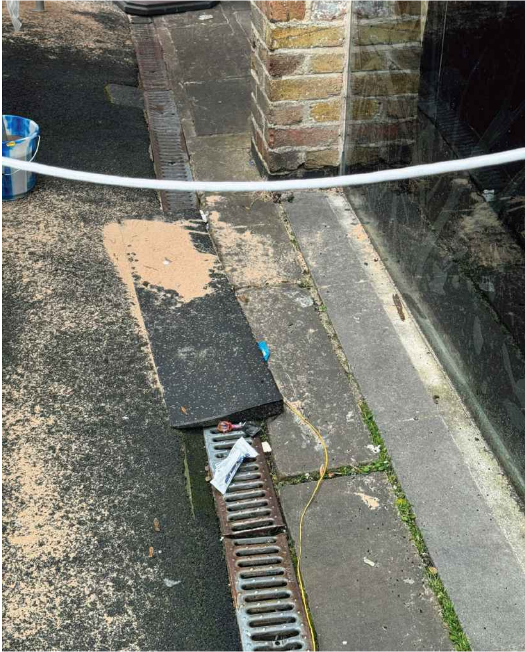
Photo 16 - Drainage along East Elvation
