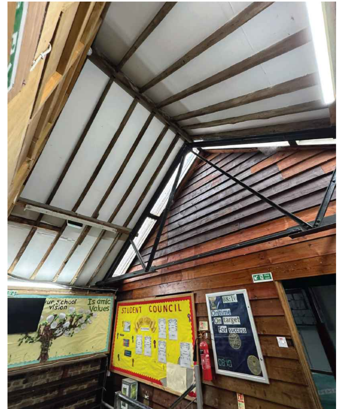
Photo 02 - North End of 19th Century Barn
