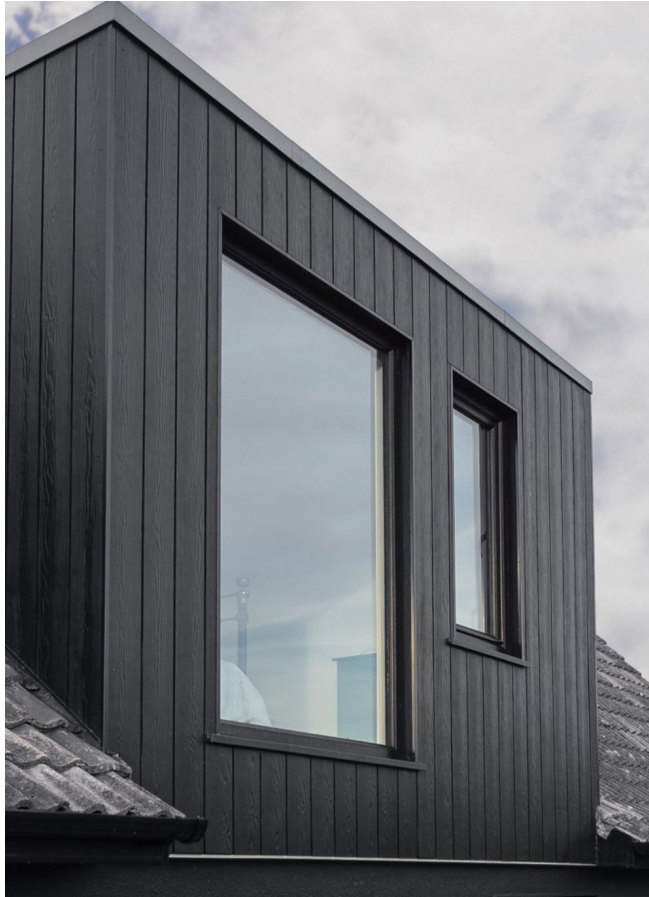
Vertical Plank Orientation, Metal Coping
