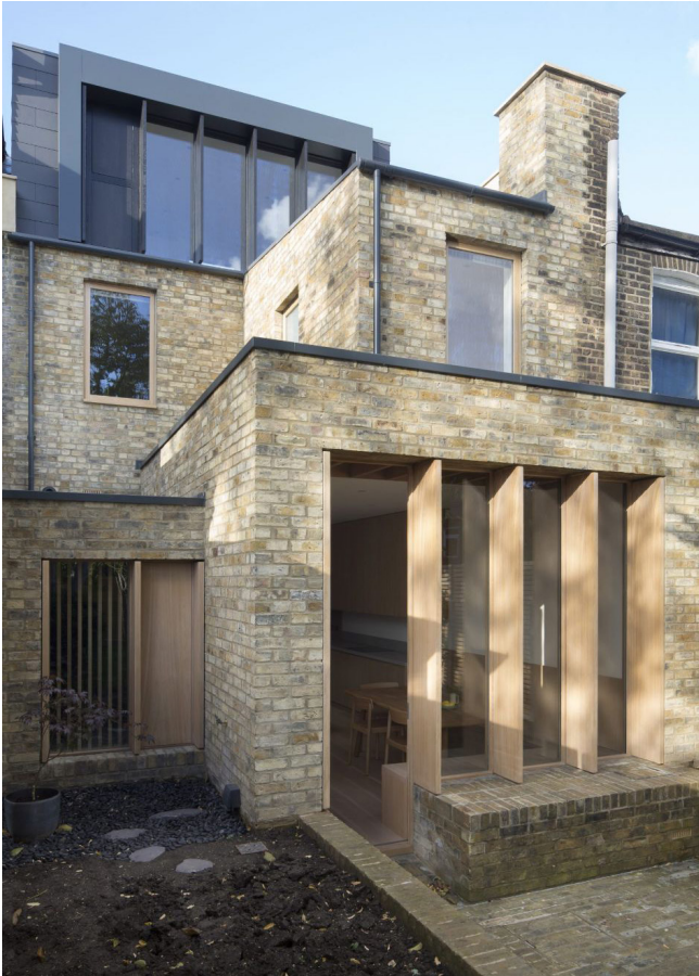
Brick Colour Matching Existing
