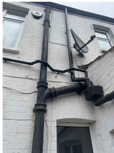
Site Photo: Rear drainage pipe locations
