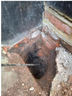
TPBH1 Excavation Probe
