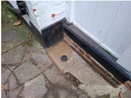
TPBH1 Completion (With Deep Datum)
