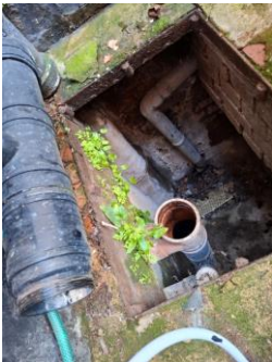
Drains Accessed for Survey
