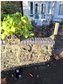
Water Meter Location
