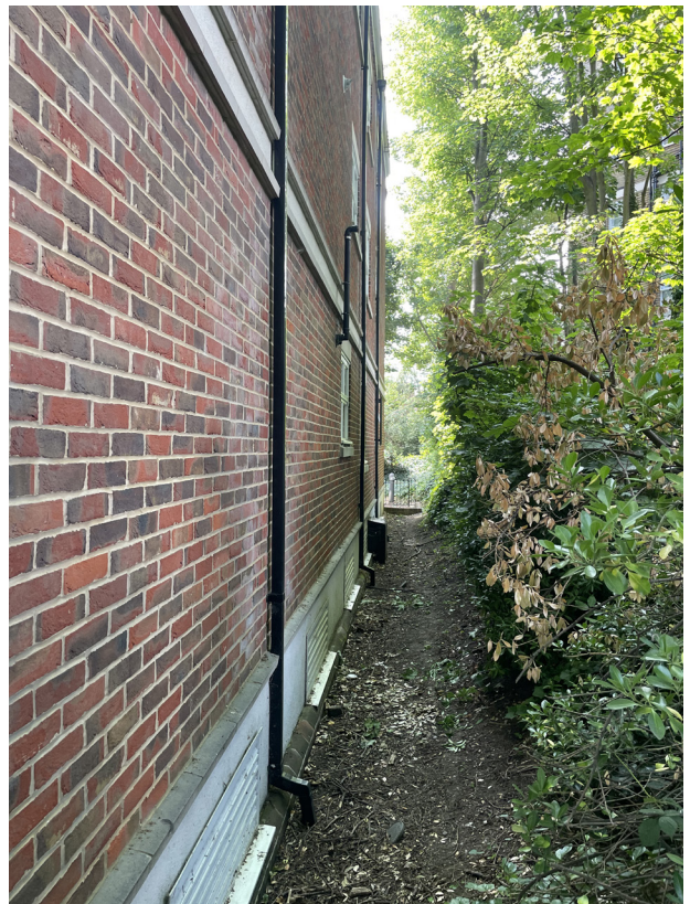
[Fig. 05] View of existing side elevation wall from the Rear Elevation.
