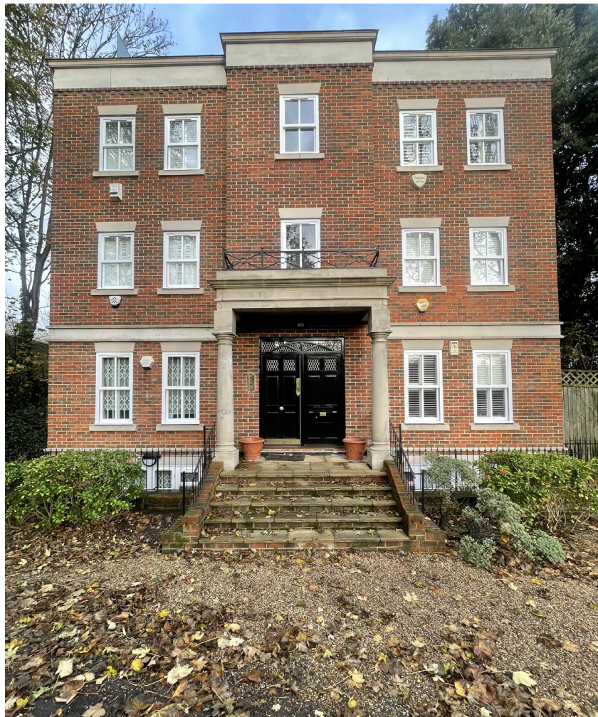
[Fig. 01] Street facing facade of Kempton House, 52 Cholmeley Park. Image from agent site visit.
