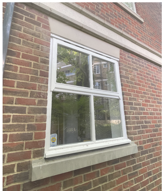
(Fig. 03) Existing sash window to side elevation Image from Agent site visit.
