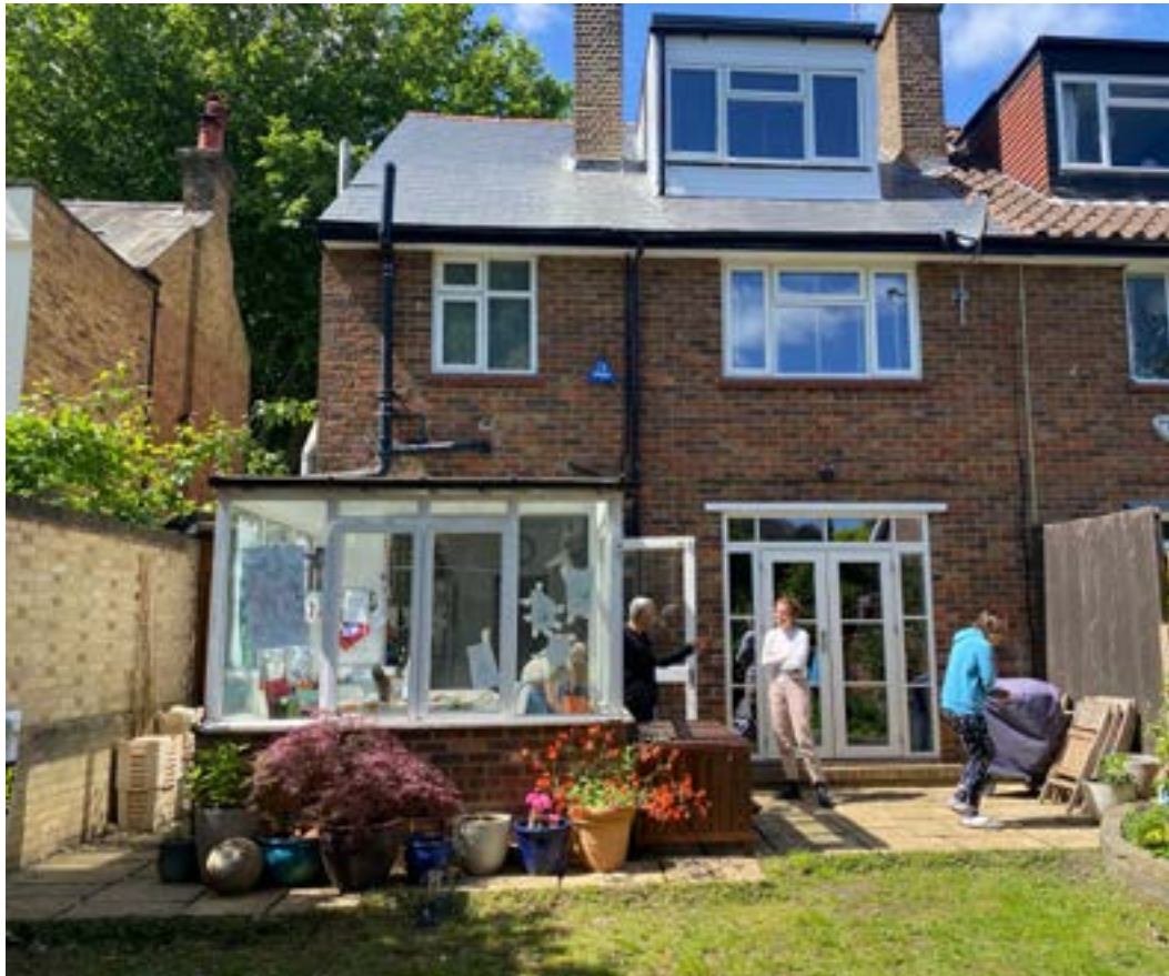
Top: View of the site, looking North from 22 North hill; Bottom Left: View of the site's rear elevation from the rear garden.
