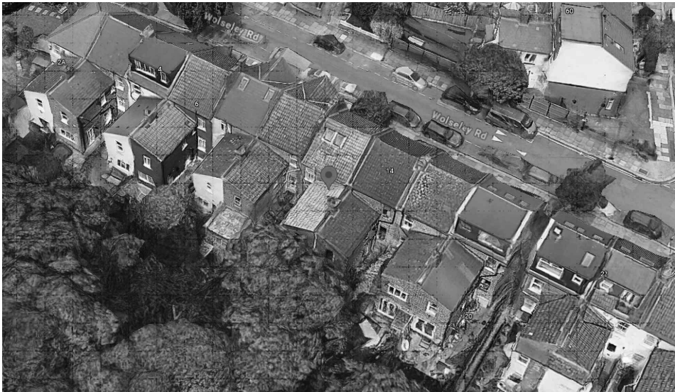
AERIAL VIEW OF EXISTING ROOFS ON WOLSELEY ROAD A MIXTURE OF CLAY TILES AND ARTIFICIAL SLATES
