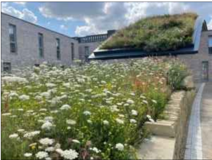
Biodiverse roof example with mixed wildflower seeding / plug plants/ Sedum planting mix with gravel finish. Log piles and rock piles to be formed in areas on the biodiverse roof.
