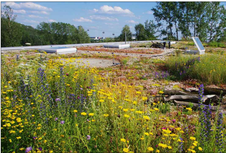
Biodiverse roof example with mixed wildflower seeding / plug plants/ Sedum planting mix with gravel finish. Log piles and rock piles to be formed in areas on the biodiverse roof.
