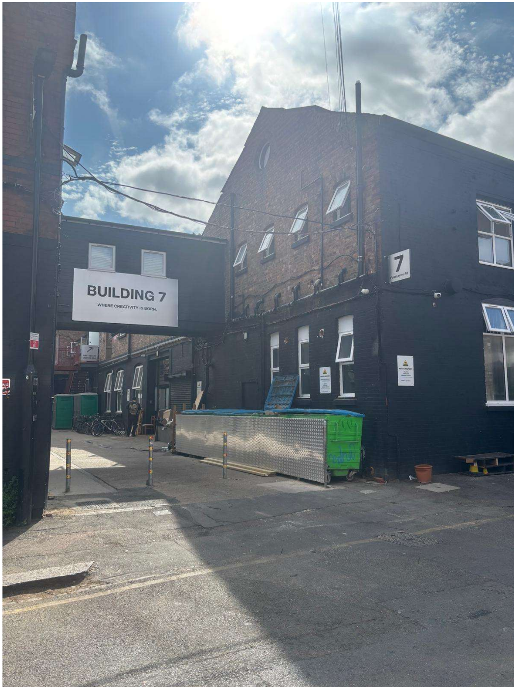
Front of the site
