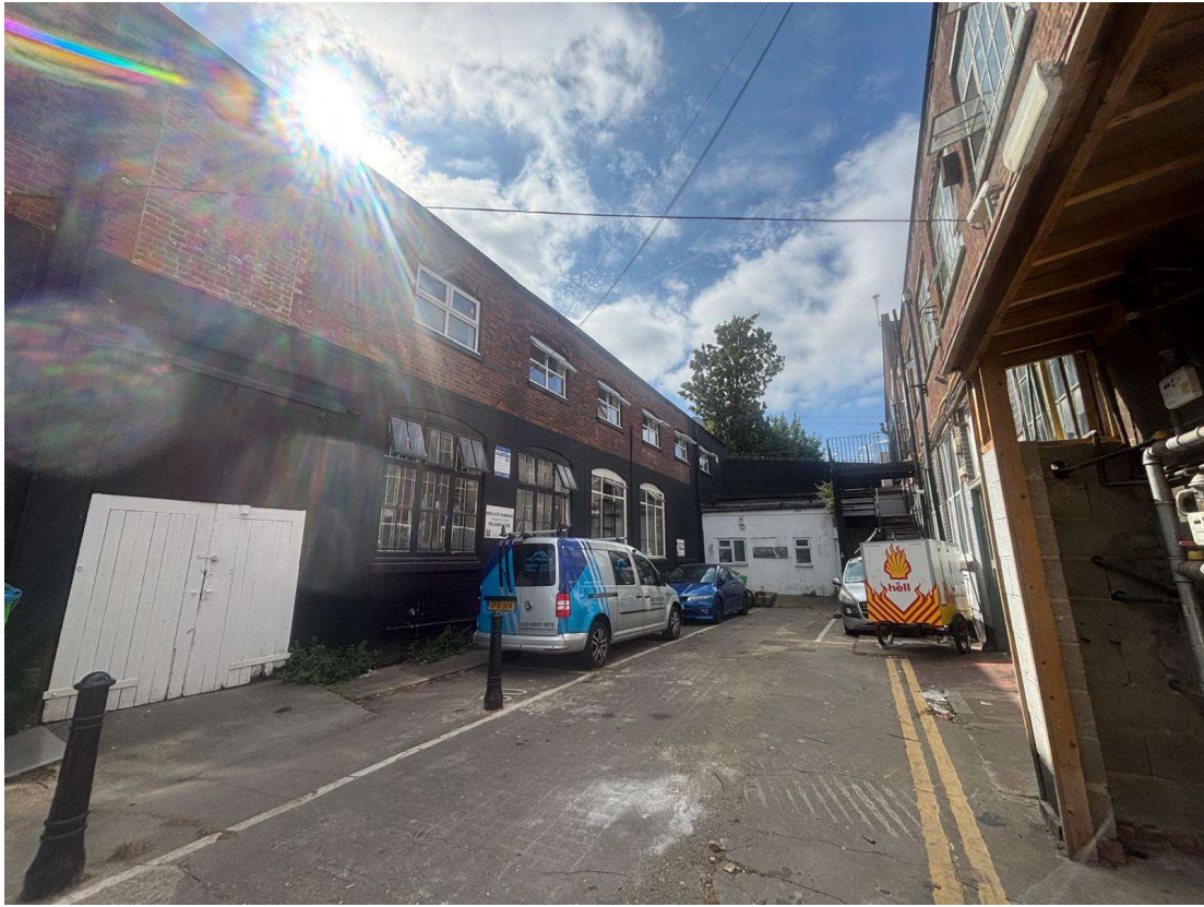
Side of the site
