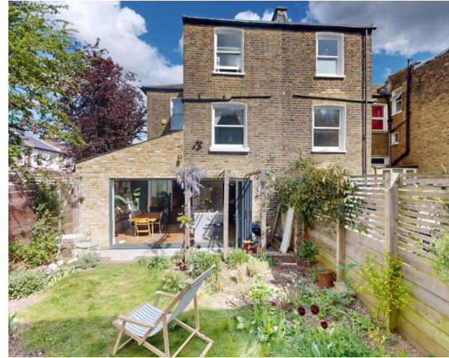
Existing Rear facade
