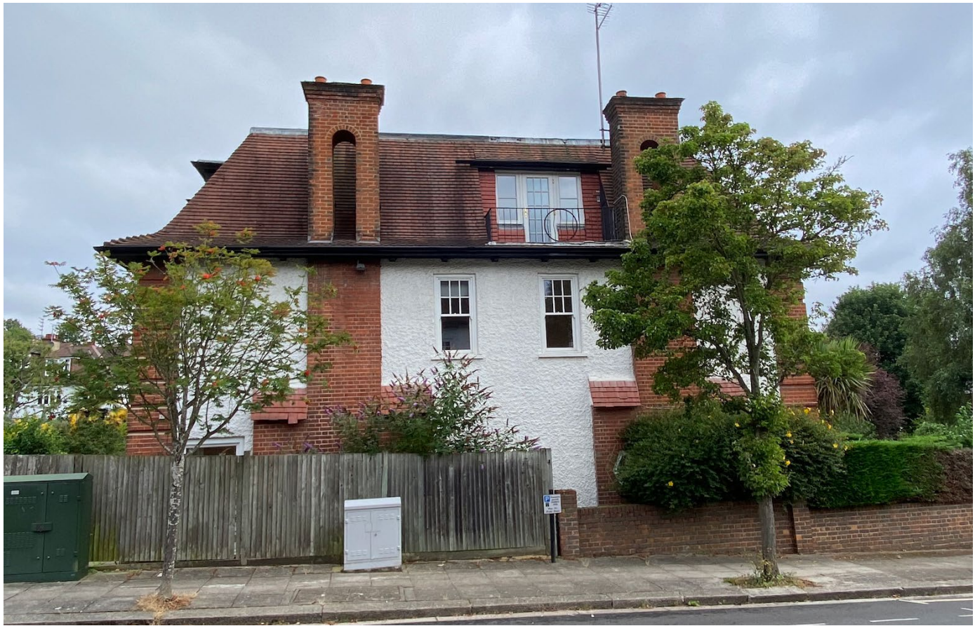
View of south side of no. 40 from Cholmeley Crescent
