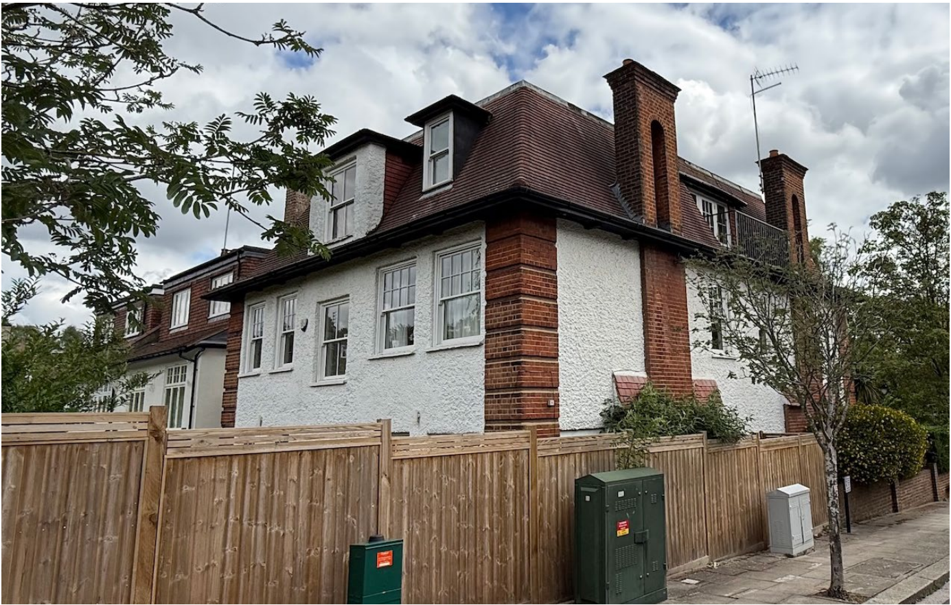
View of rear of no 40 from Cholmeley Crescent
