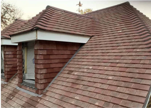
DORMER TILES TO MATCH EXISTING ROOF TILES
