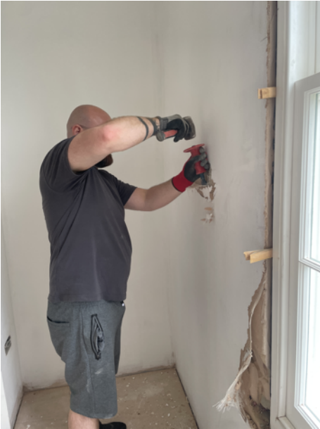
Carefull removal of gypsum plaster using hand tools
