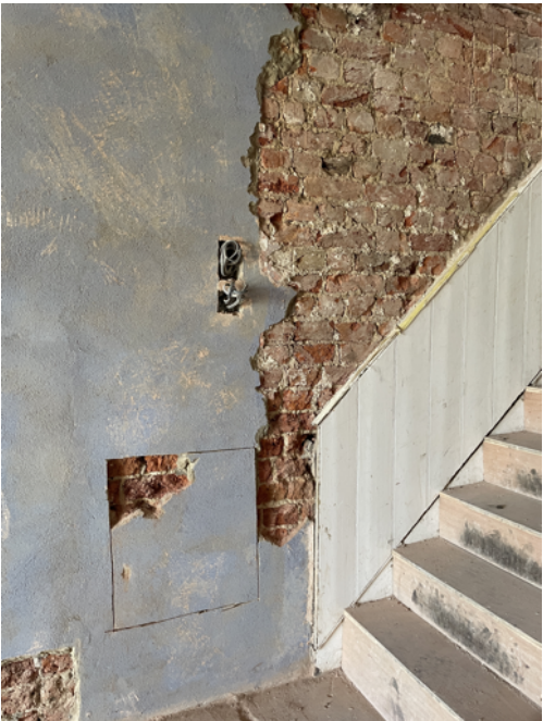
Existing panelling to LGF stair
