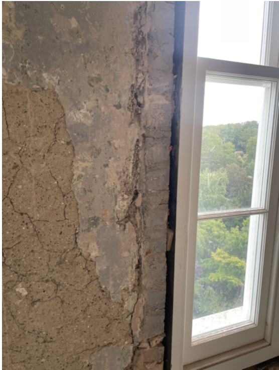
Window junction detail to 2nd floor where architrave needs packing out to allow for full depth of plaster
