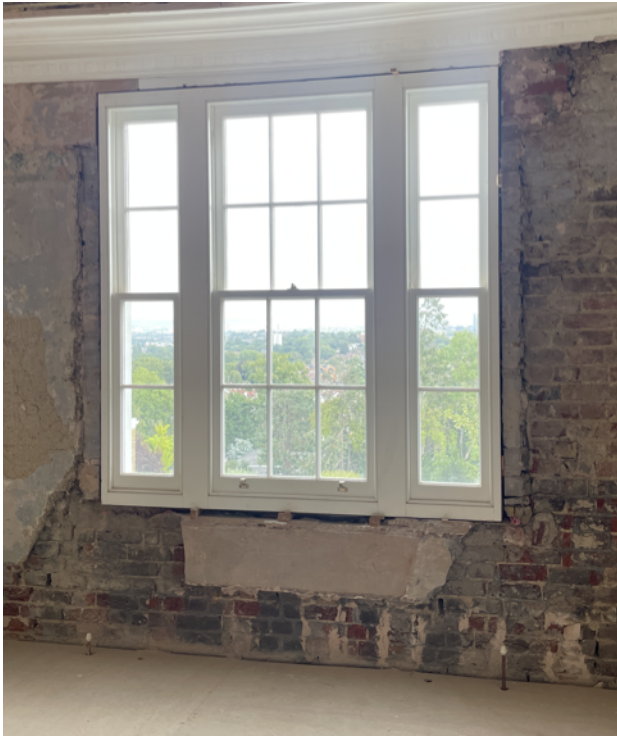
Window junction detail to 2nd floor where architrave needs packing out to allow for full depth of plaster
