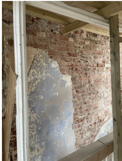
First floor hallway party wall
