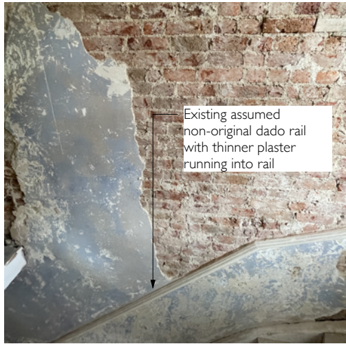
Existing dado rail on Ground to 1st Stair
