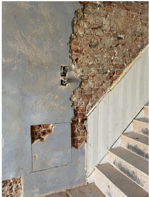
Existing panelling to LGF stair
