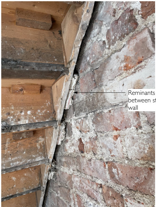
Underside of existing ground to 1st floor stair
