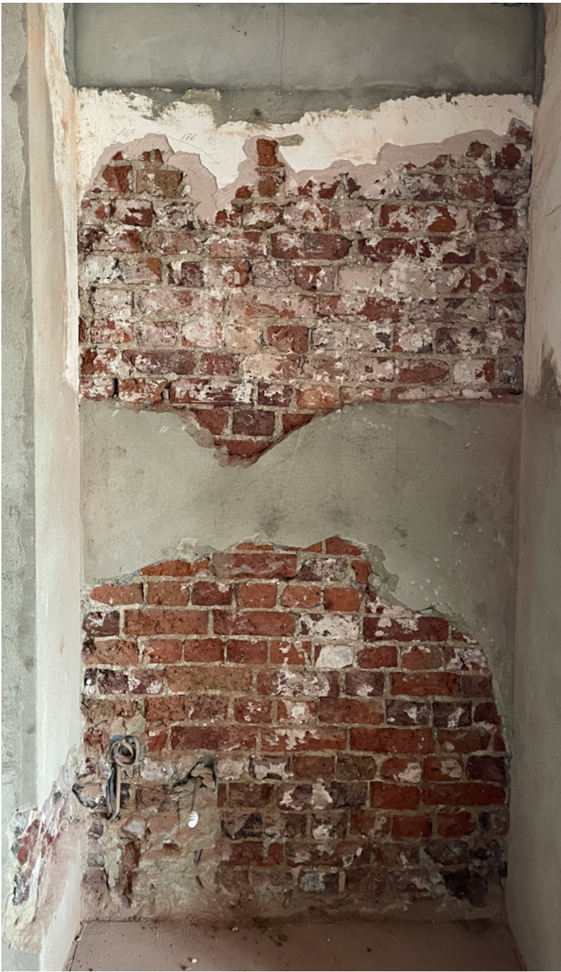
N5 - Trial areas to northern wall with varying damage. Upper render removes more easily with little damage to brick. At lower levels more damage is present with brick faces coming away, but the bricks remain stable. Render removal to continue carefully. Where removal causes more extensive damage localised areas of render will be retained
