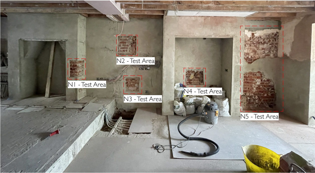
Northern wall test areas
