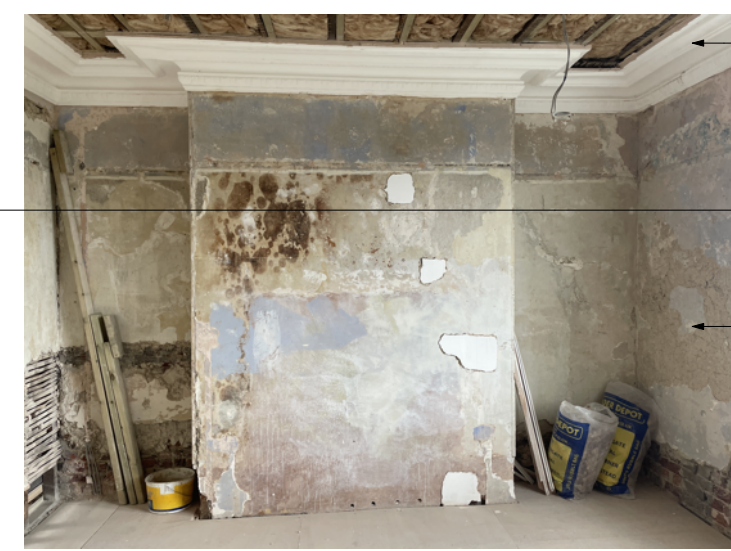
Second Floor Rear Room
