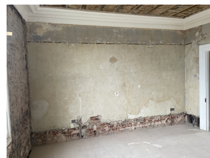
Second Floor Rear Room
