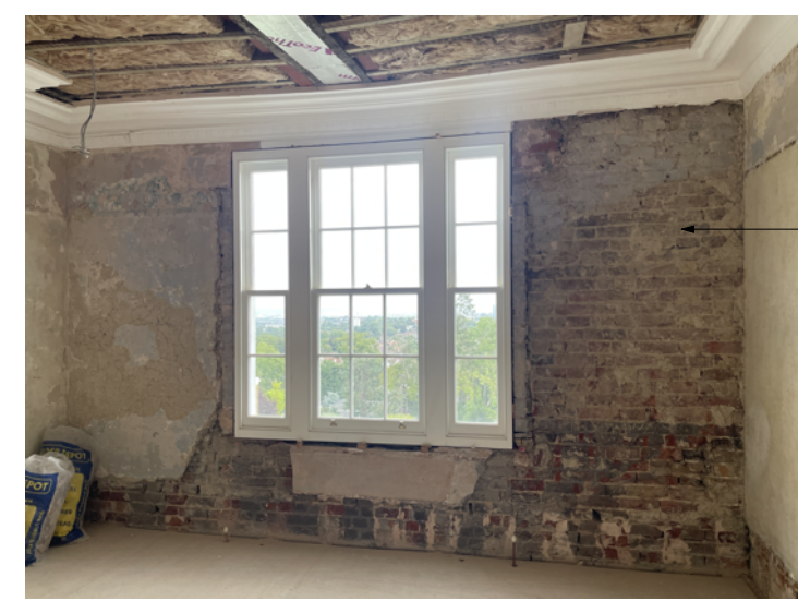
Second Floor Rear Room
