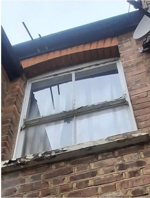
Rear First Floor Window
