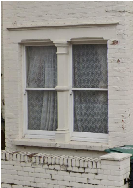
Front Ground Floor Window
