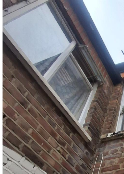
Rear Side First Floor Window
