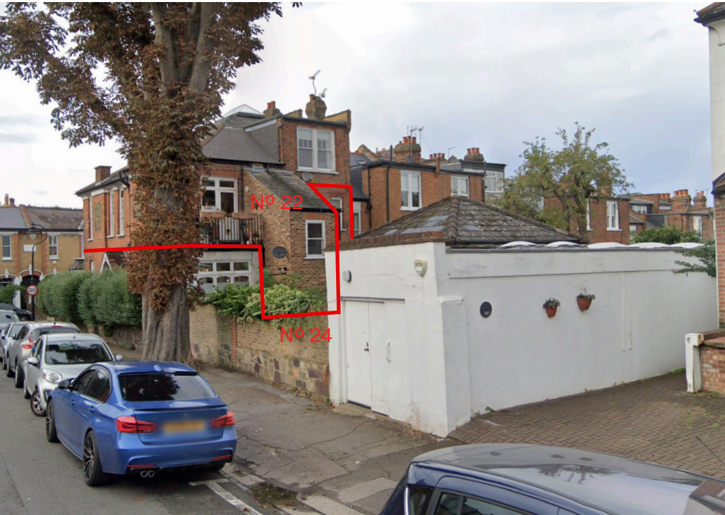
Front View (Source Google Maps). A semi detached house split into 2 properties.
