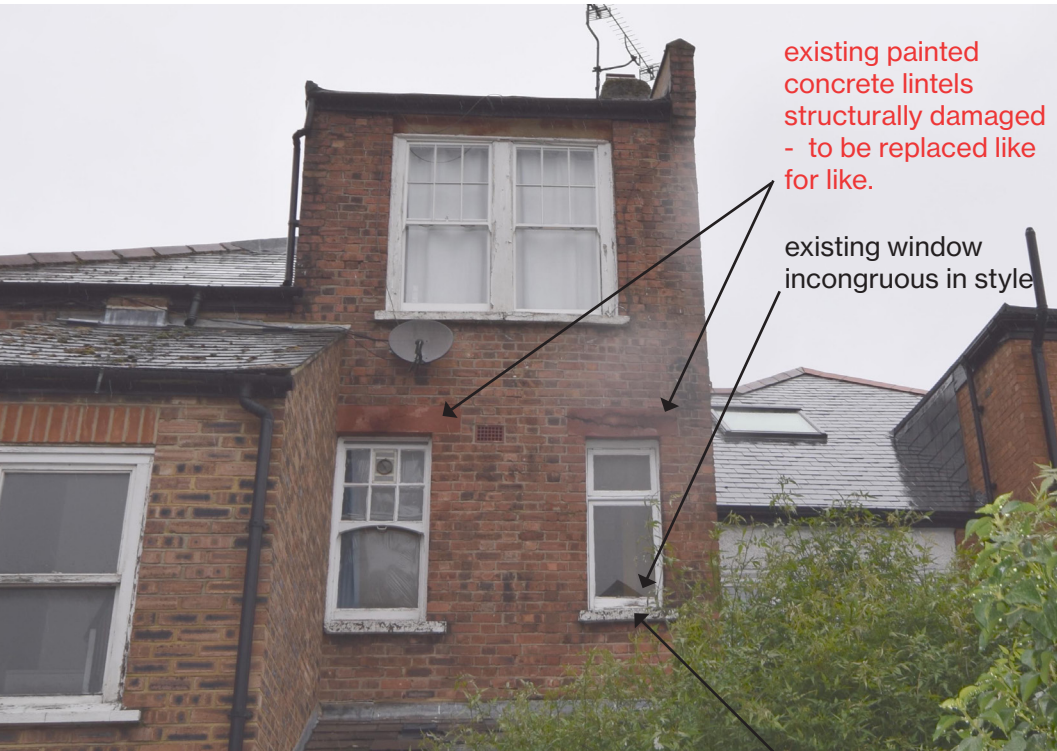
Side passage (similar down both sides of property).
