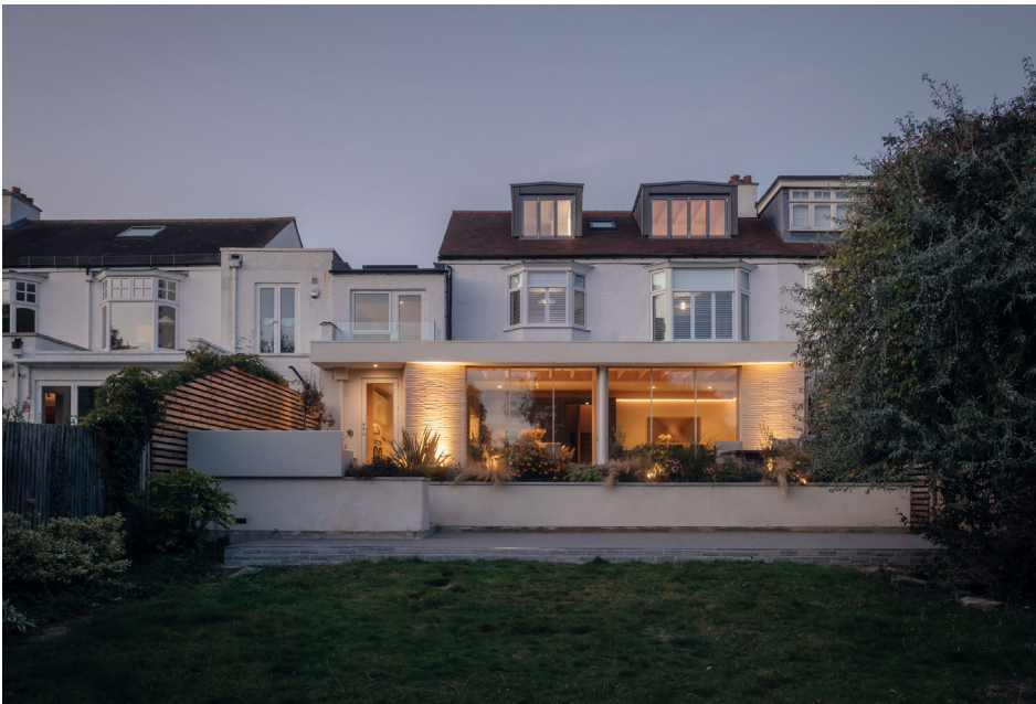
Dulwich Park House, LB Southwark & Dulwich Estate, 2024.
