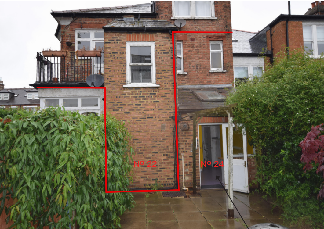
Rear View - Stepped rear elevation
