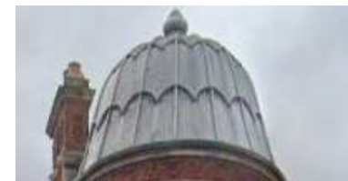
Lead roofing
