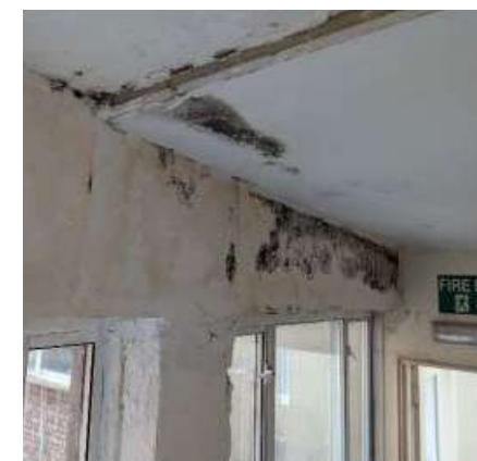
Damp and mould present above some windows at upper levels. Some partition walls and finishes are in poor condition with visible holes
