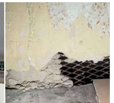
Damp and mould present above some windows at upper levels. Some partition walls and finishes are in poor condition with visible holes
