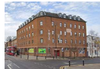
Re-clad with roof extension 1980's
