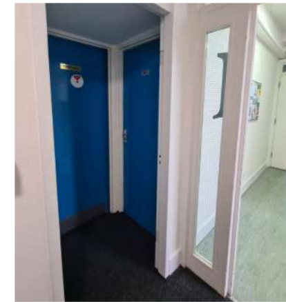
Narrow corridors to bedrooms and some rooms directly accessed from core lobby which could potentially pose fire and safety risk hazard
