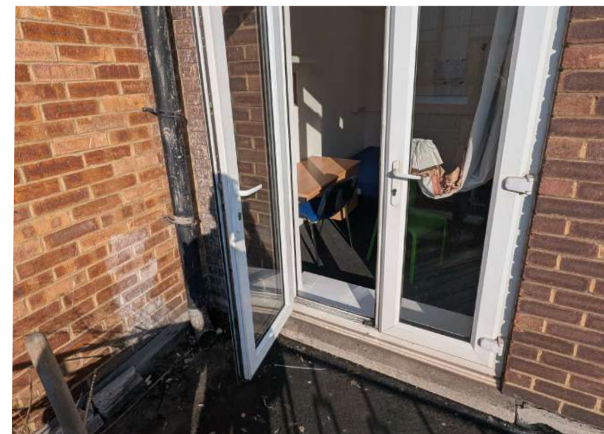
Windows to first floor bed spaces along Tottenham Lane. Windows are placed on restrictors and kept locked for safeguarding purposes
