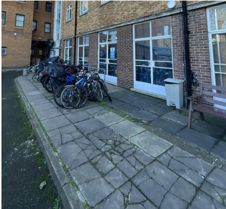
Figure 7: Concrete paving slabs in the yard.
