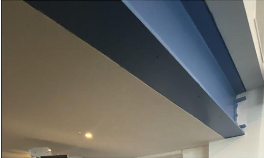
Figure 8: Exposed structural steel beam in the Fitness Centre.
