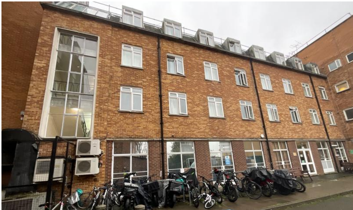
Figure 11: Exterior of the site showing exposed brick.
