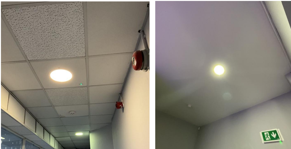
Figure 10: Gypsum ceiling tiles, and plasterboard wall and ceiling finishes in the Fitness Centre.
