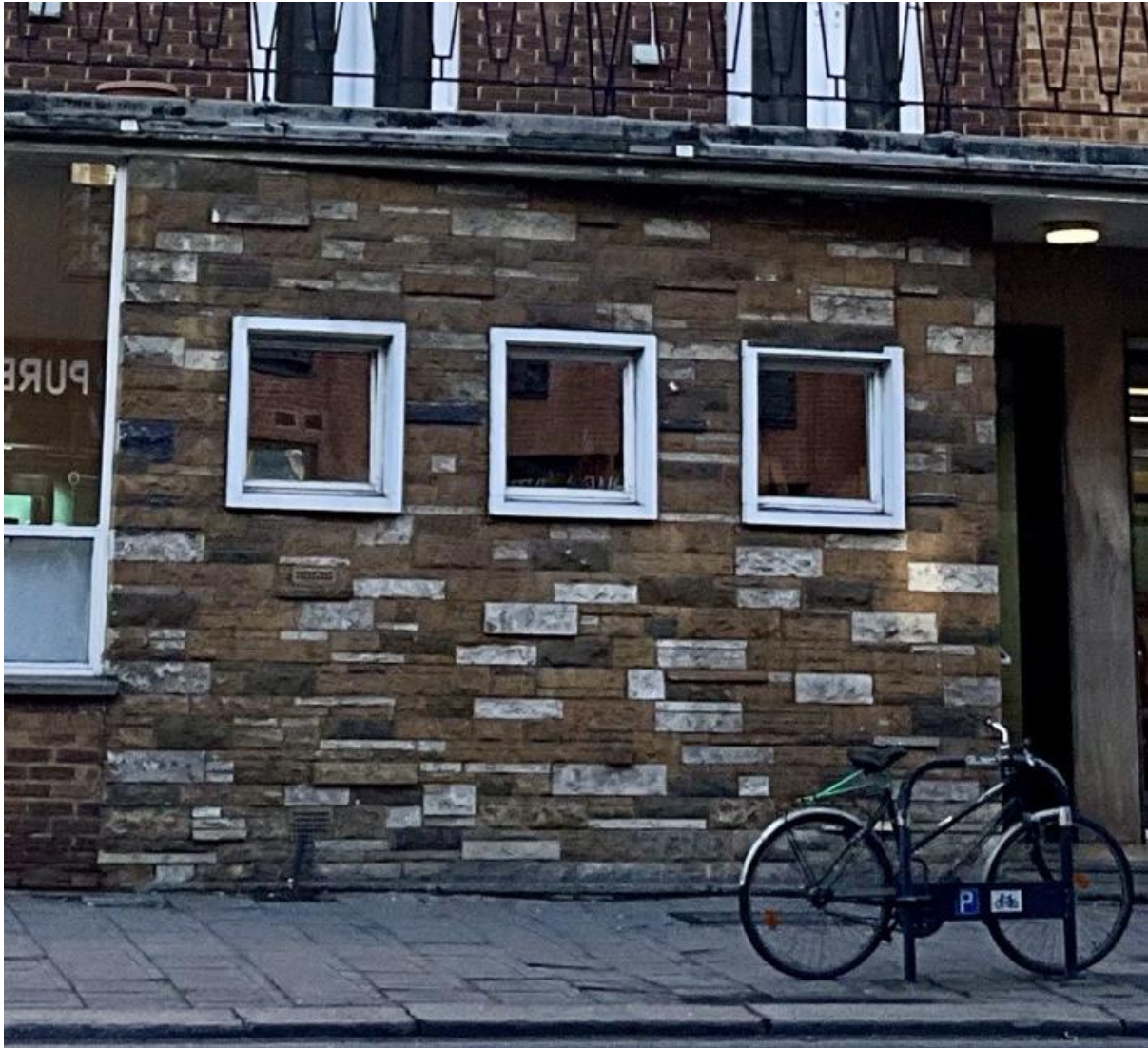
Figure 12: Stone cladding on the Sir Brett Cloutman Wing façade
