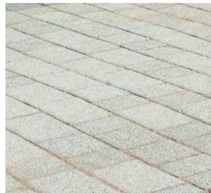
Concrete sett paving to circulation spaces
