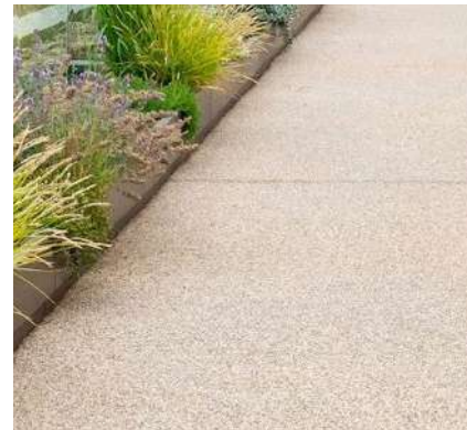
Permeable resin-bound gravel to courtyard activity zone
