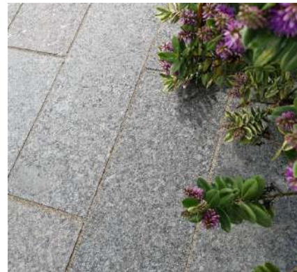
High-quality paving to key building entrances
