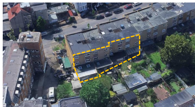
Figure 16: 49-55 (odd) Rosebery Gardens windows
