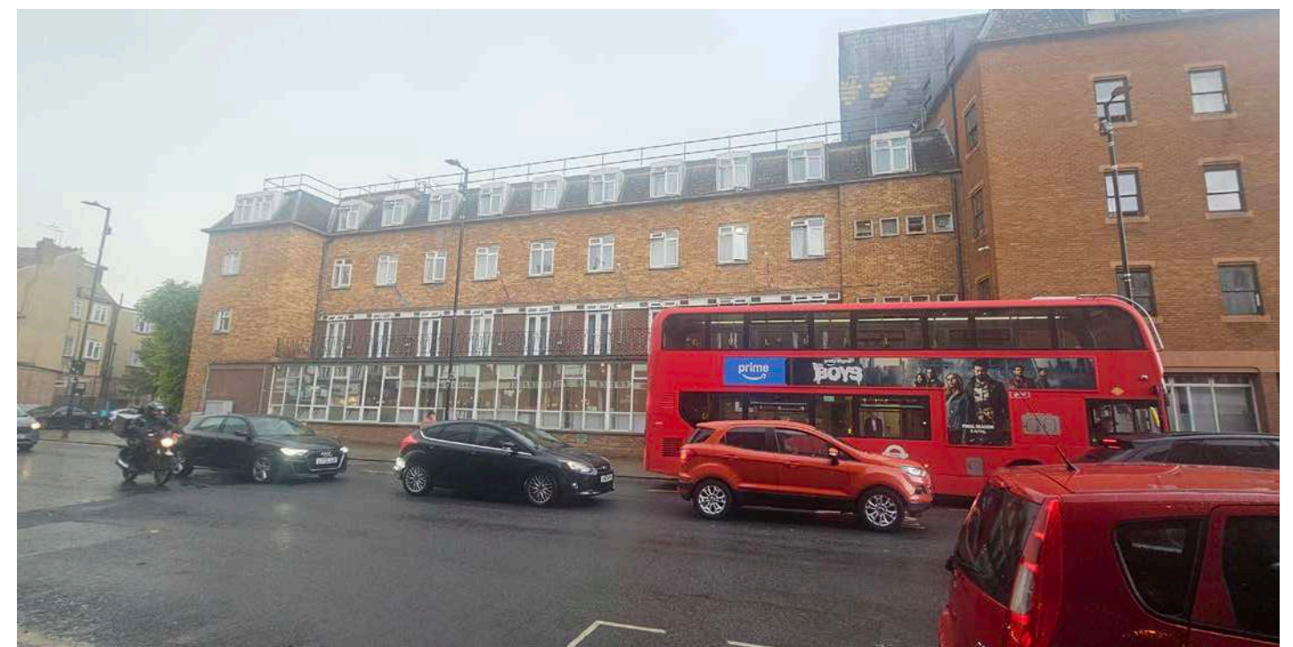
Figure 1.3 The Site from Tottenham Lane - Site Visit 2026
