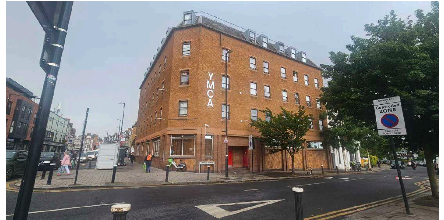
Figure 1.2 The Site from the Corner of Tottenham Lane and Elmfield Avenue - Site Visit 2026
