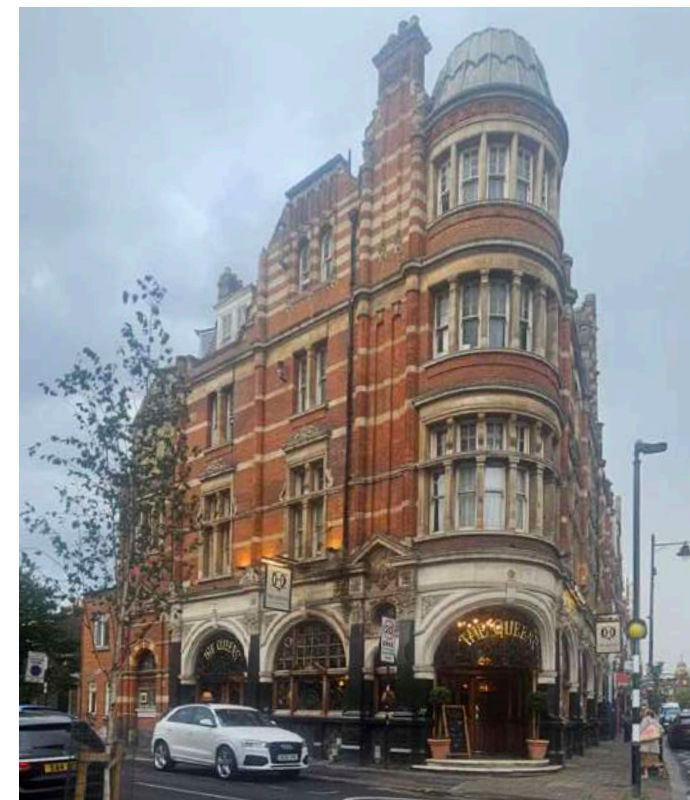
Figure 3.30 The Queens Public House - Site Visit 2026
