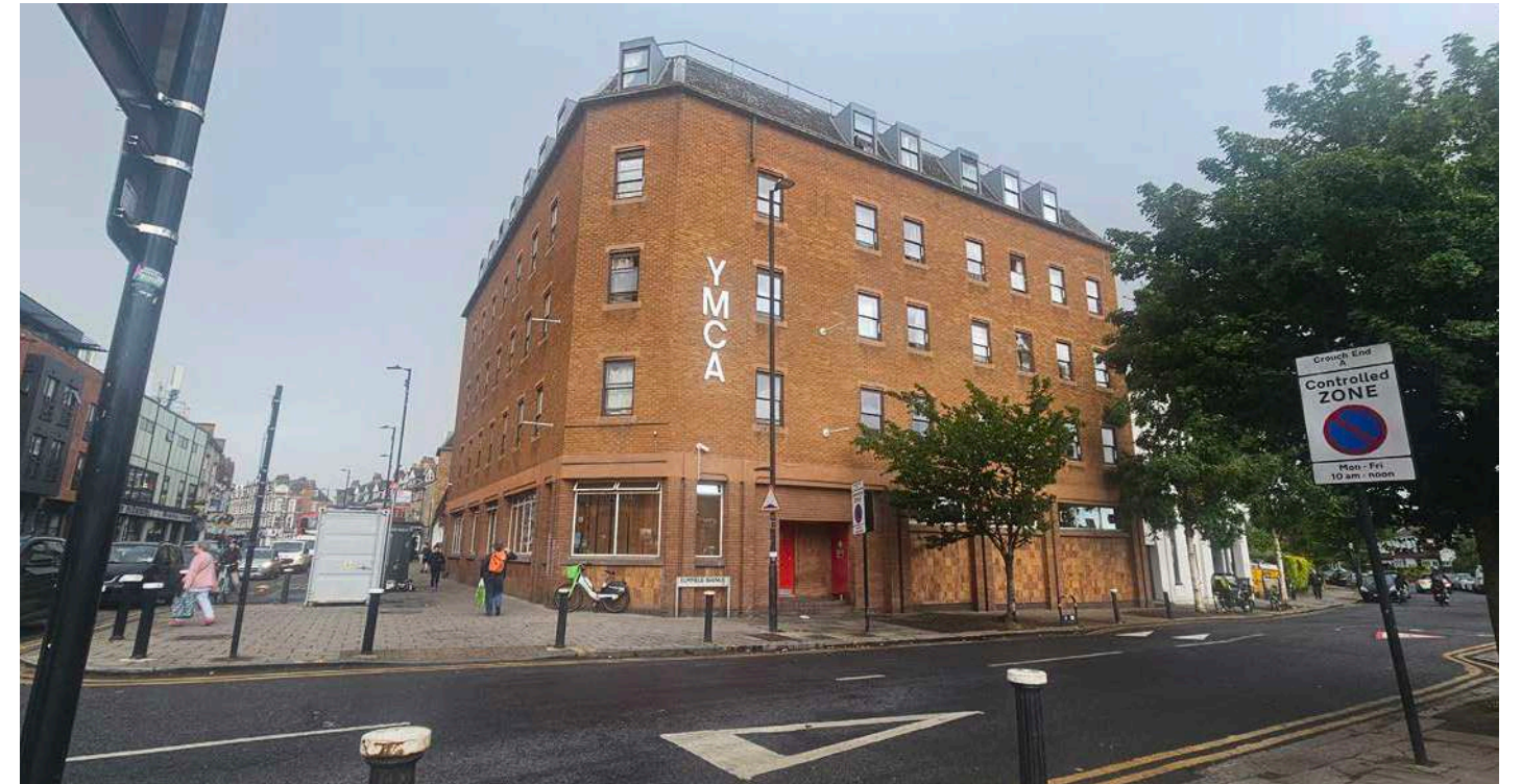
Figure 3.39 The Site View from Elmfield Avenue of the main elevation - Site Visit 2026
