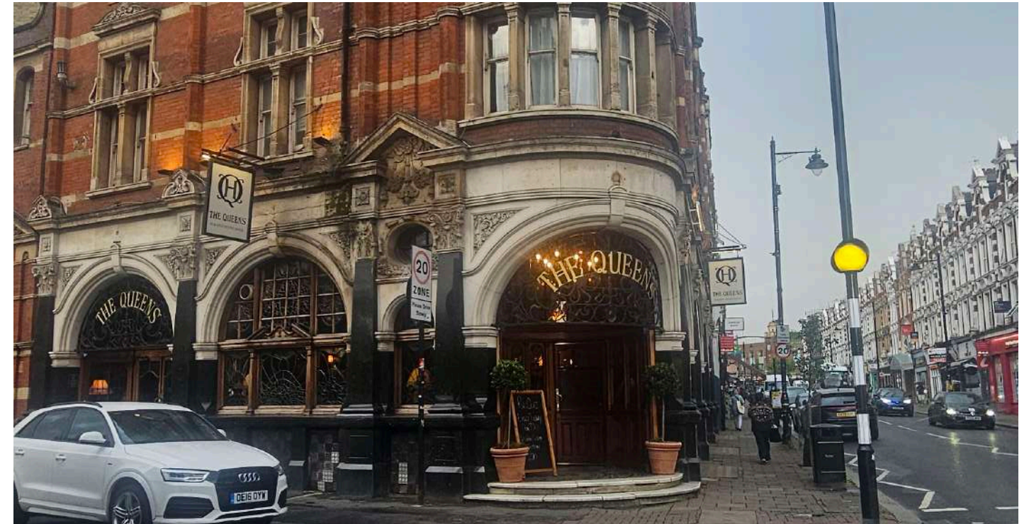
Figure 3.28 The Queens Public House - Site Visit 2026
