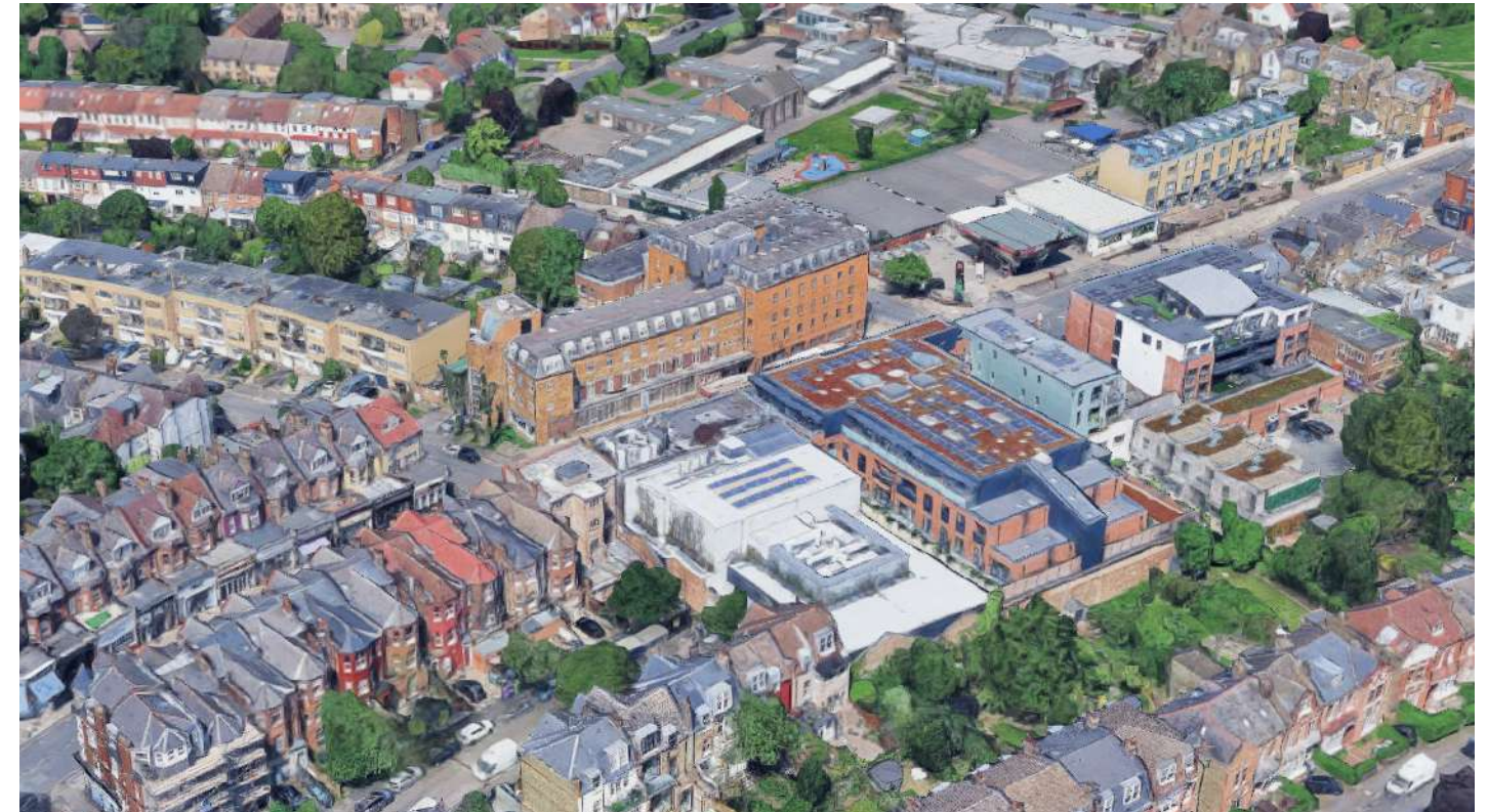
Figure 4.13 Aerial view Google Maps 2026 - 5. Larger Scale Civic and Commercial Buildings Character Area
