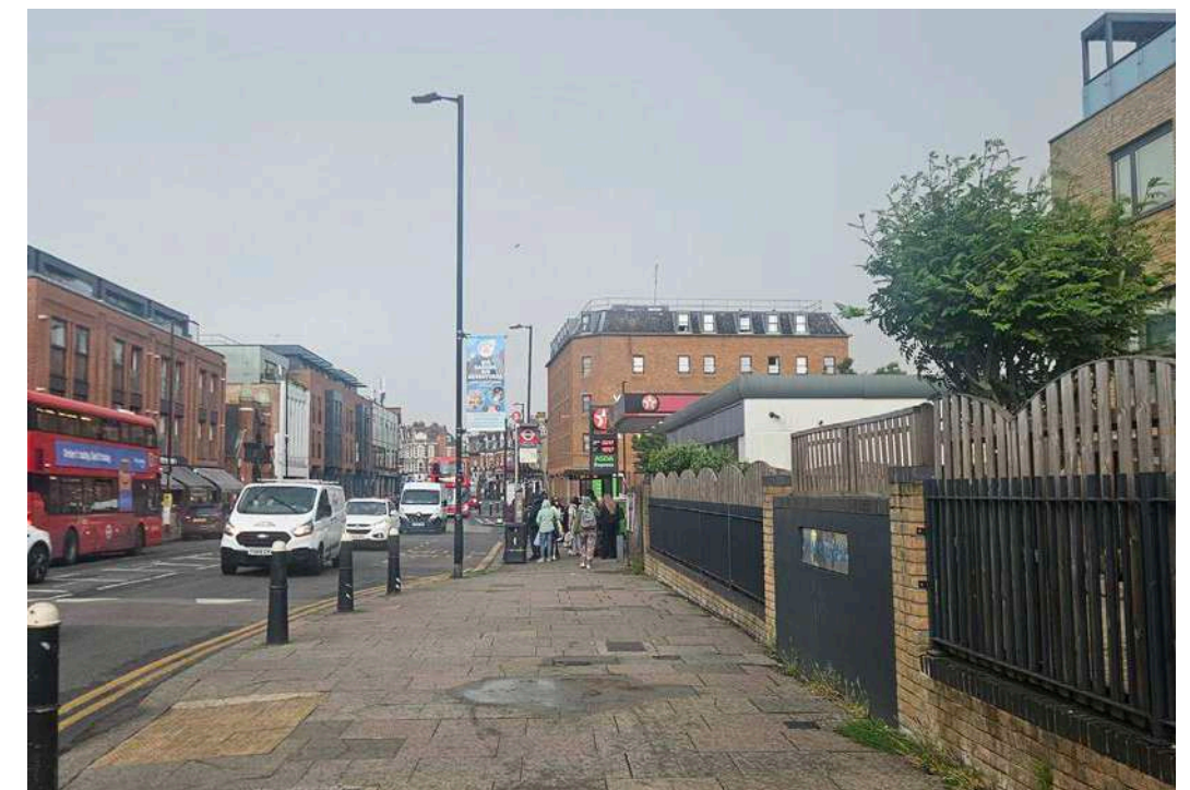
Figure 4.14 5. Tottenham Lane - Larger Scale Civic and Commercial Buildings
