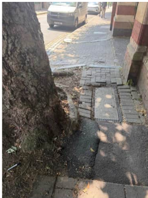
Figure 4-6: ATZ Route 3 – Worst Point – Tree Root Growth on Footway of A1201 Crouch Hill
