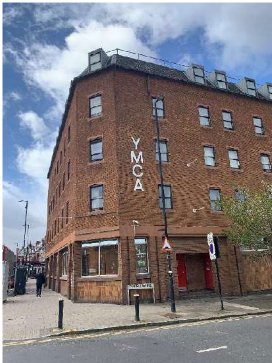
Photograph 7: South eastern corner of building
