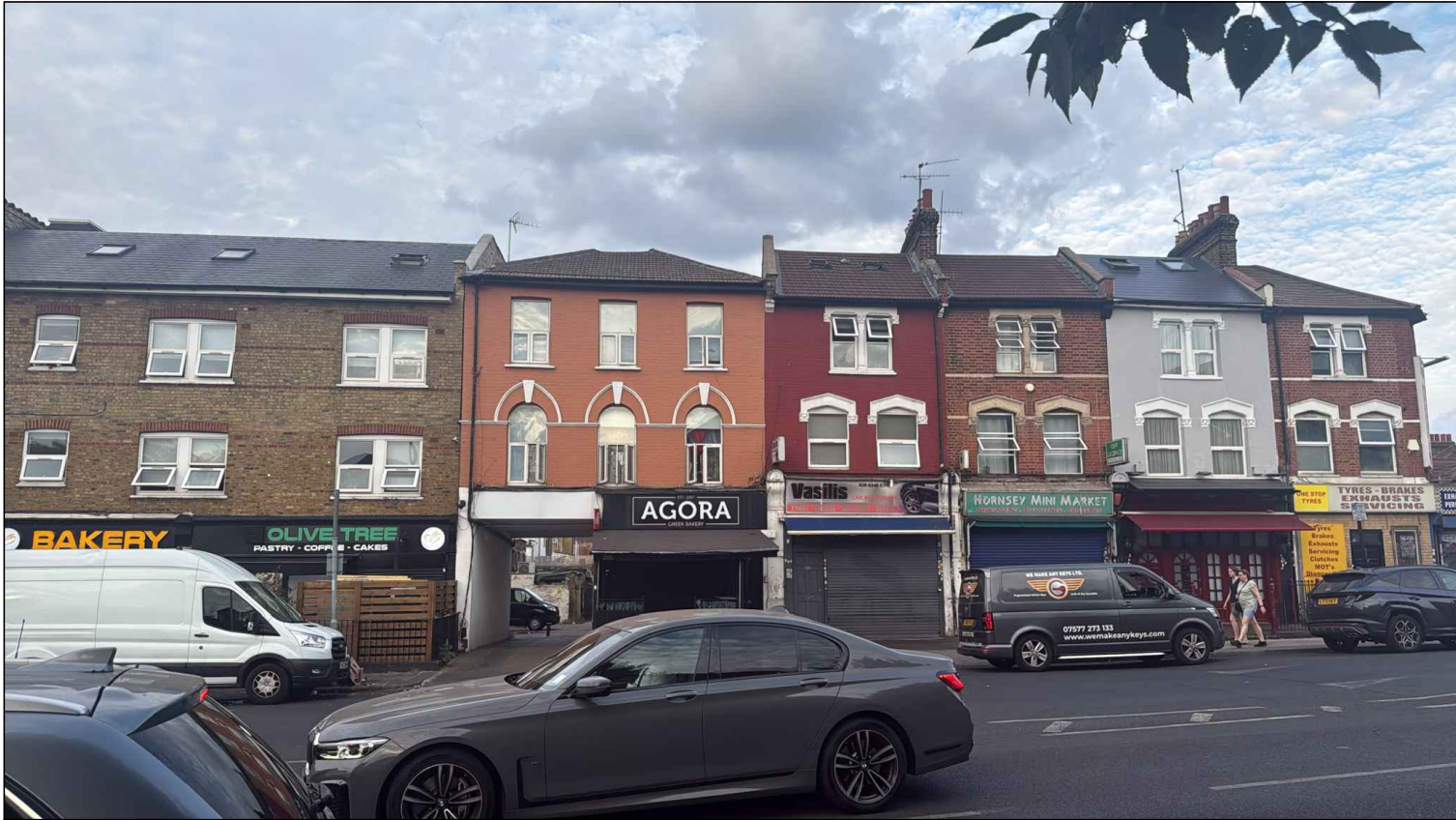
STREET VIEW 2 AS EXISTING
