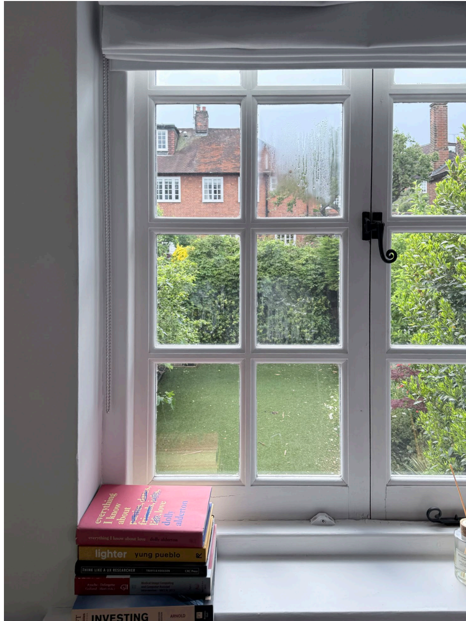
1. Existing slimline double glazed timber windows in rear elevation.
