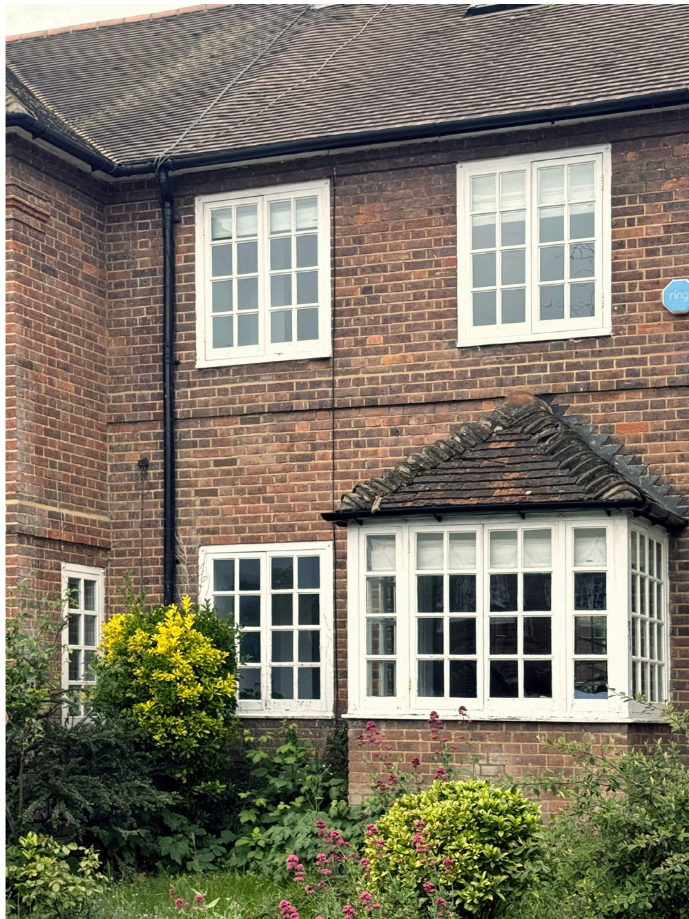
1. Mixture of single glazed and slimline double glazed timber windows.
