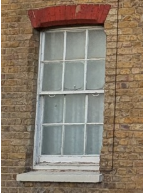
Front Elevation Ground Floor Window (East)
