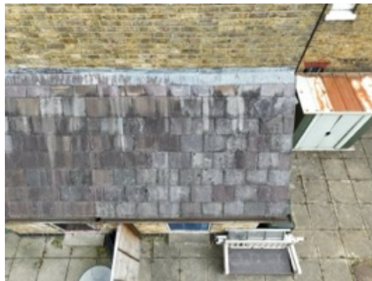
Existing Rear Lean-to Roof
