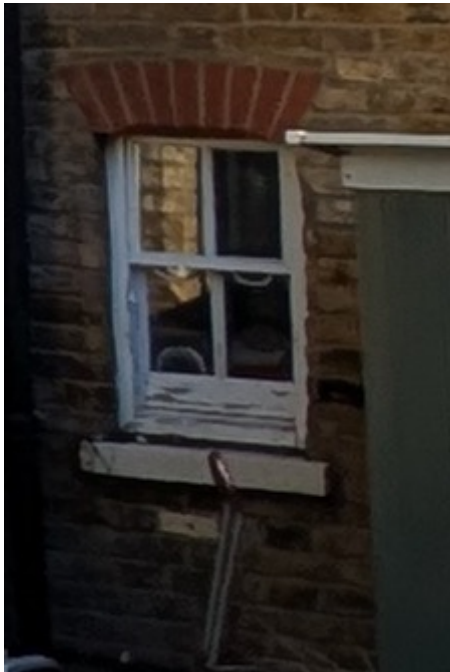
Rear Elevation Ground Floor Window (West)
