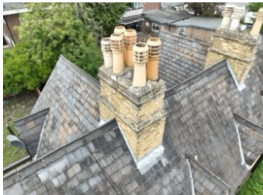
Existing Roof Chimney's
