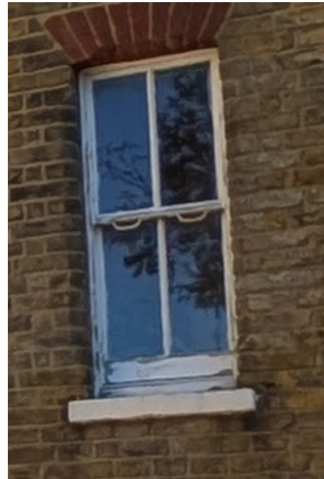
Rear Elevation First Floor Window (West)
