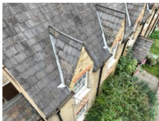
Existing Roof Gables
