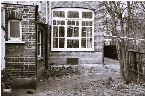
View 4 before scaffolding
