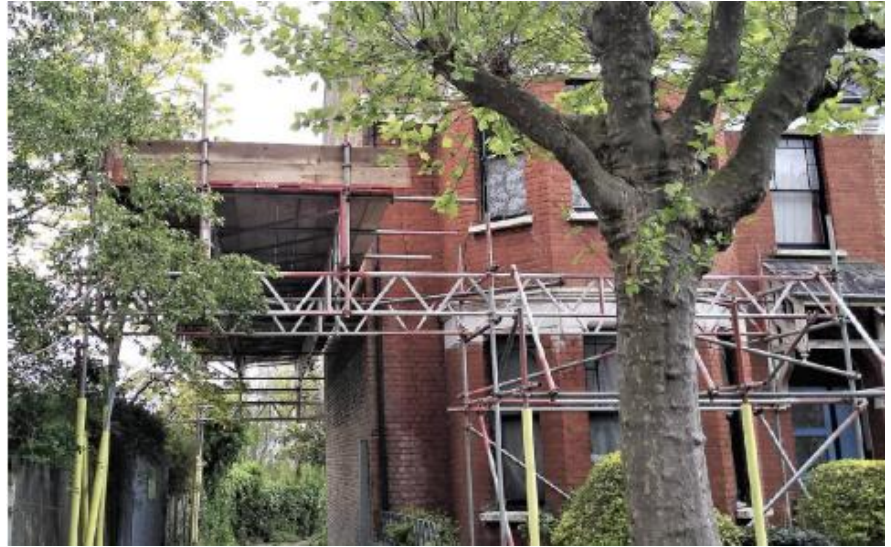
View 1 with crash deck scaffolding
