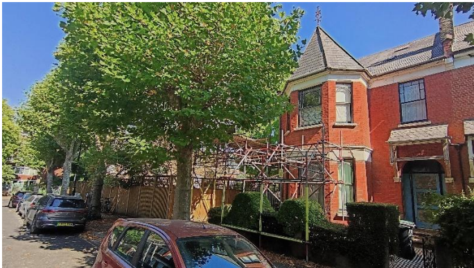
View 2 with scaffolding
