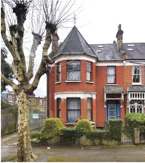
View 1 before scaffolding
