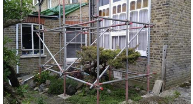
View 5 with scaffolding
