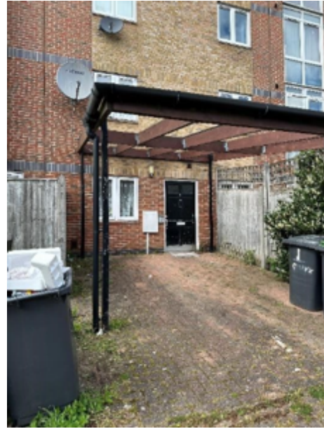
Flat One Entrance Door
