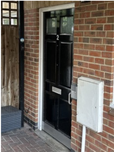
Flat Two Entrance Door
