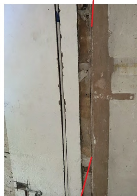
EVIDENCE THAT INTERNAL STUD PARTITIONS ARE RECENT AS MODERN PLASTER BEHIND
