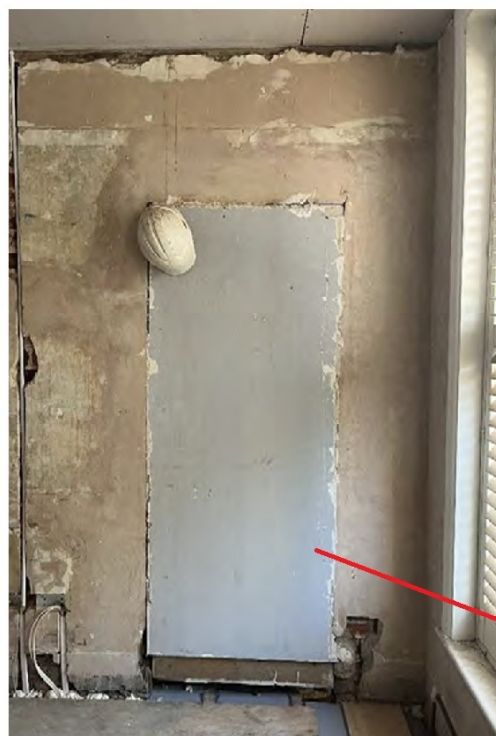
EVIDENCE OF FORMER DOOR OPENING TO NEXT DOOR
