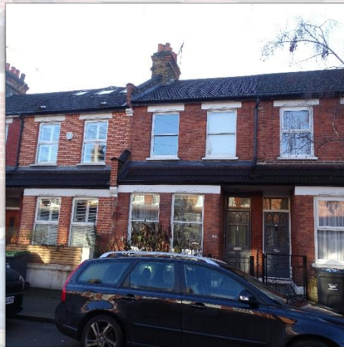
Above: View of the front fenestration of 40 Falmer Road
