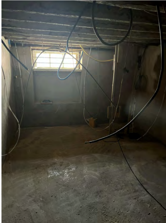
Plate 11 – View through the basement towards the front elevation.
