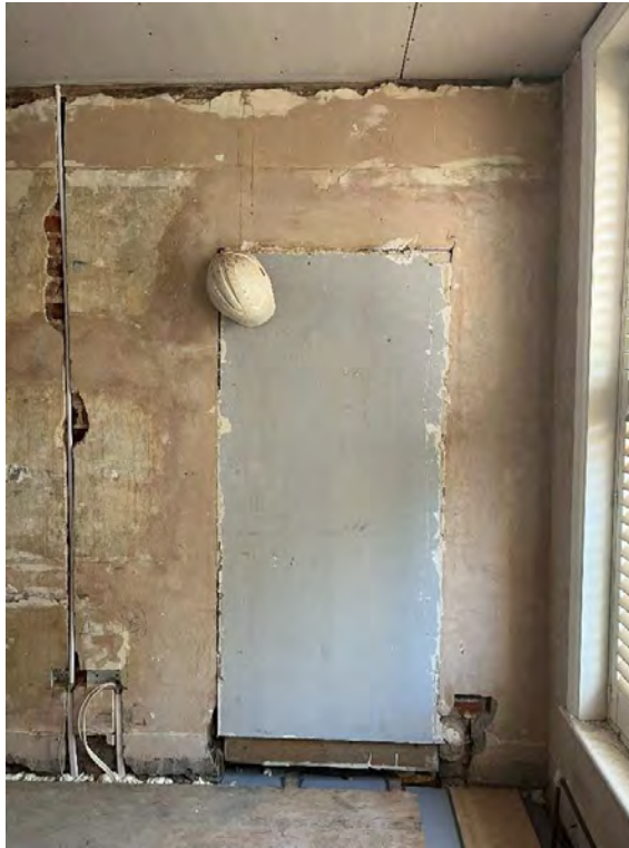
Plate 19 – Infilled door opening with the internal east wall with No. 82.
