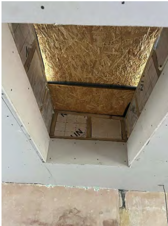
Plate 24 - Existing roof window within the renewed flat roof covering.
