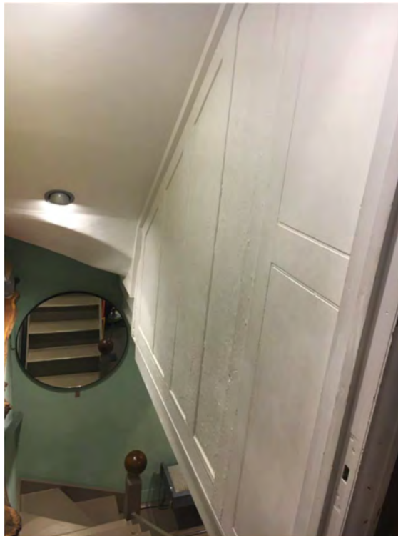
Fig 3 – Copy of image showing reinstated panelling to the lower staircase between the basement and ground floor included within the 2020 DAS.
