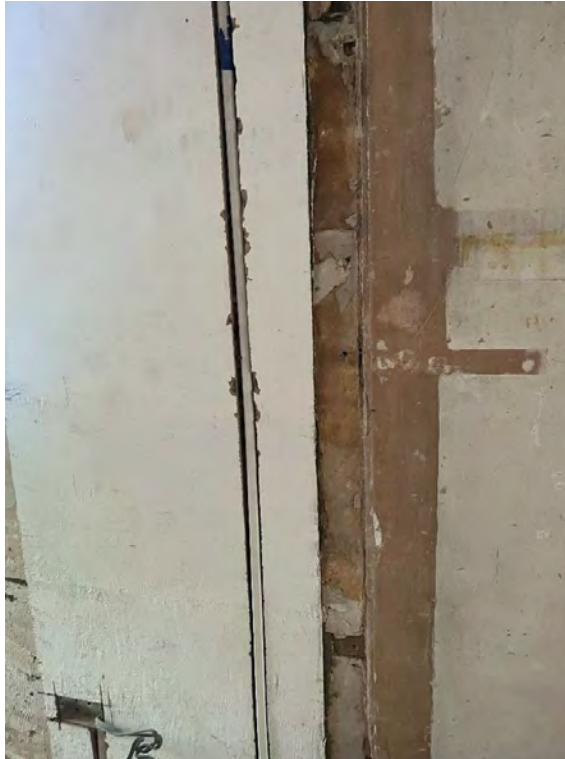
Plate 25 - Modern plaster behind where a stud partition has been removed.
