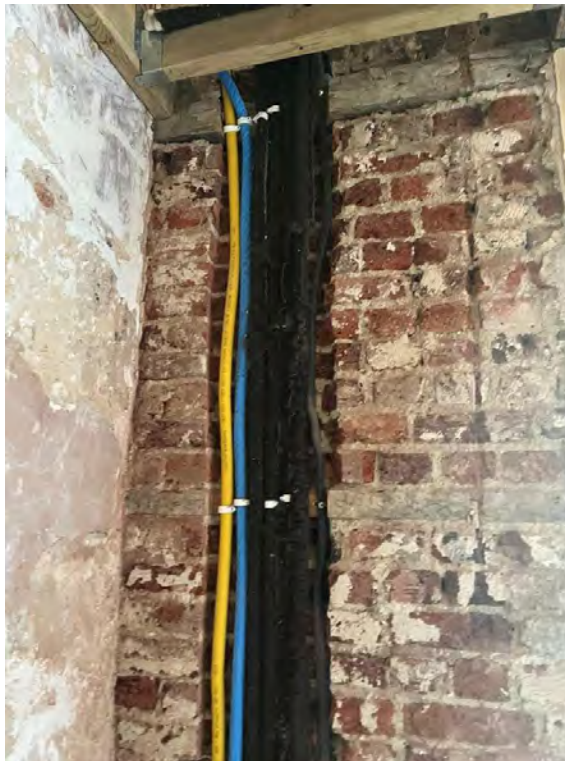
Plate 18 – Existing channel in brickwork in the rear wall reused for accommodating services.
