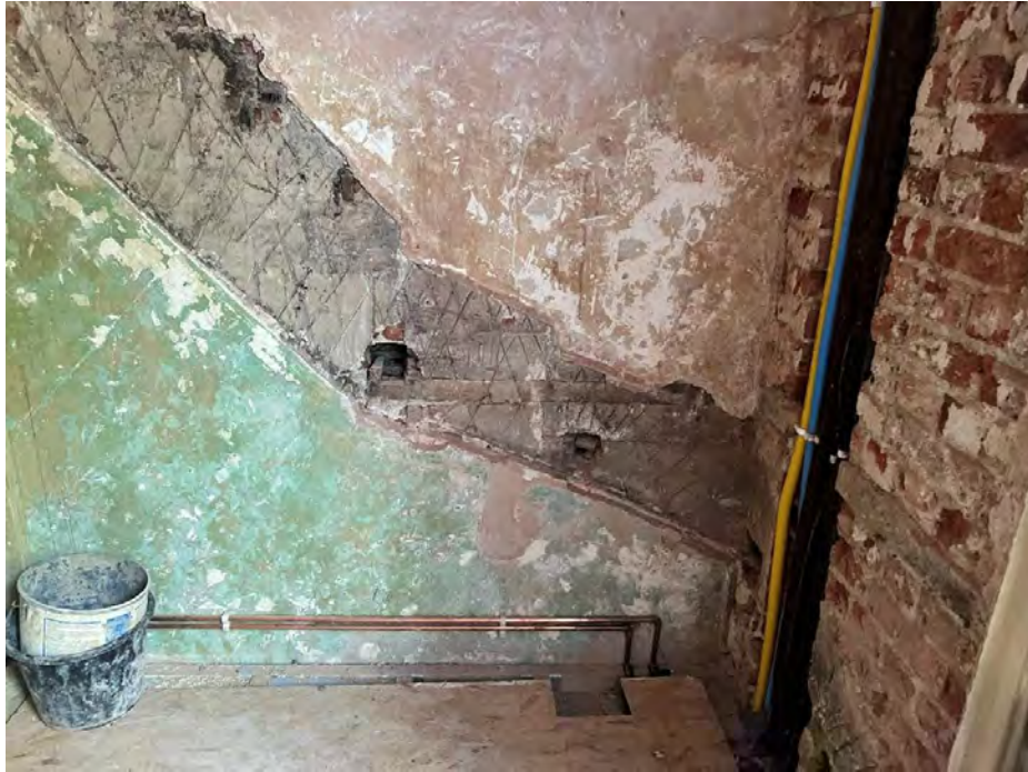
Plate 17 – Position of previous staircase with modern cement render behind where it was installed.
