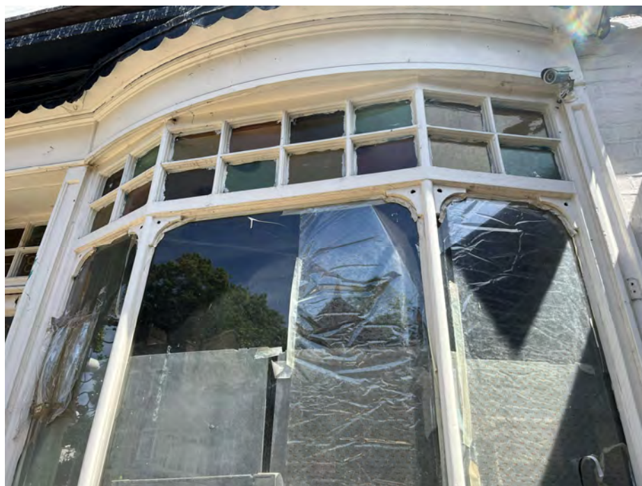
Plate 4 – Shop frontage detail.
