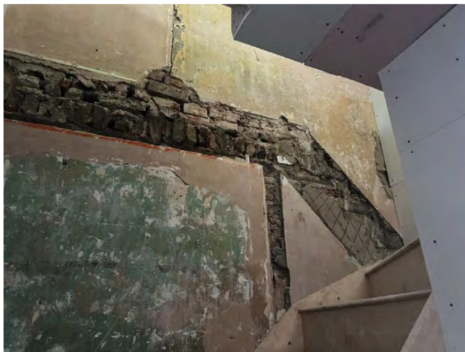
Plate 22 - Evidence of previous staircase at second floor level with modern render behind where the staircase was attached.
