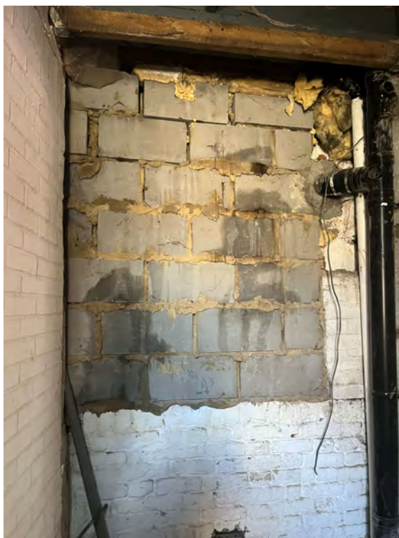
Plate 8 – Blockwork infill to the east side of the rear infill extension.
