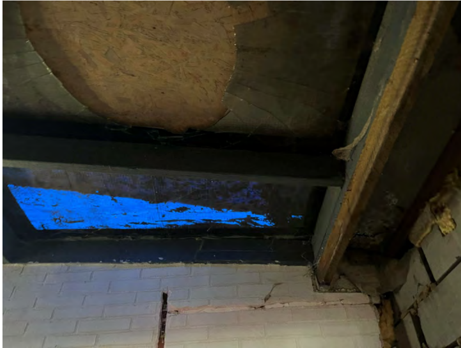
6.4 Plate 9 – Roof structure to the infill extension; solid and glazed panels proposed to be replaced with insulated glazed panels.
