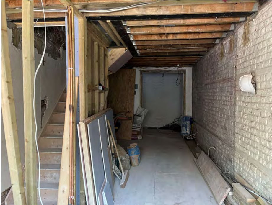
6.5 Plate 13 - View through the ground floor shop unit towards the rear elevation.
