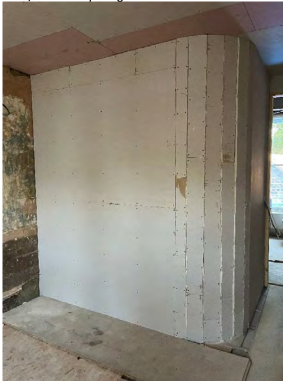
6.6 Plate 20 – New fire-rated stair enclosure to the first floor.
