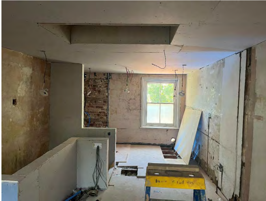
Plate 23 – View through the second floor looking towards the rear elevation.
