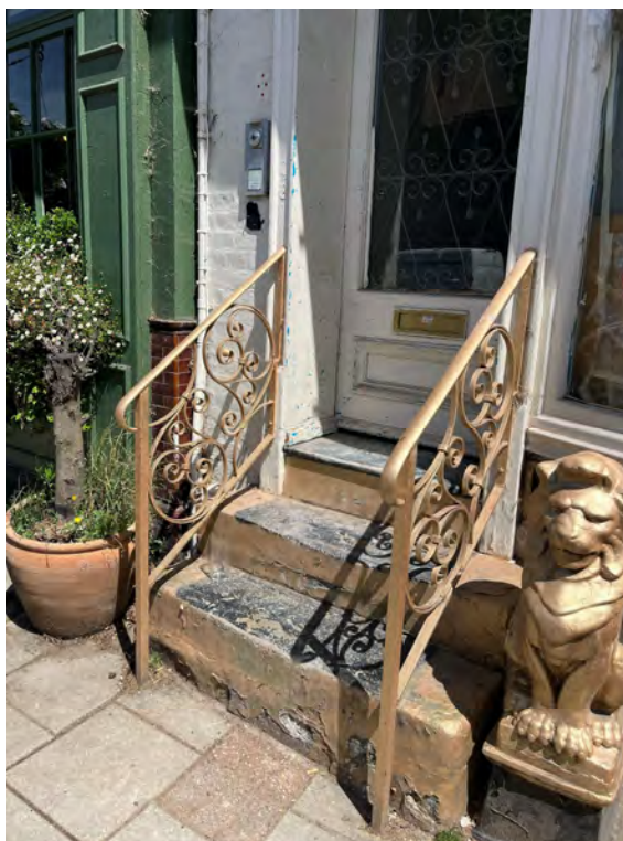
Plate 3 – Decorative cast metal balustrade to the entrance steps.
