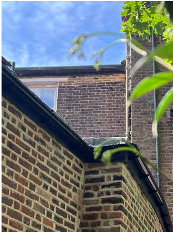
Plate 6 - Rebuilt upper courses of brickwork to the rear elevation.
