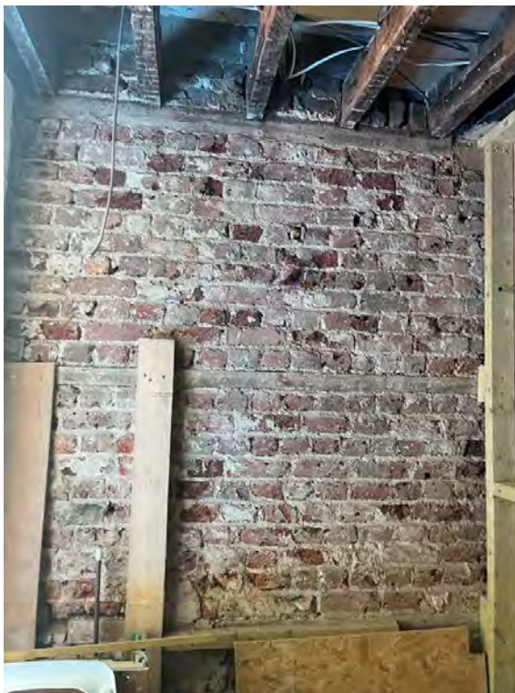
Plate 27 – View of the east internal wall; no service installed here to minimise disturbance to historic fabric.
