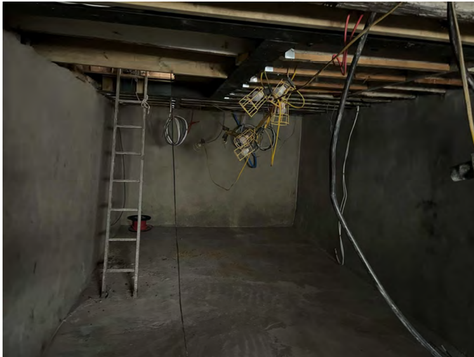
Plate 10 – View through the basement towards the rear elevation.
