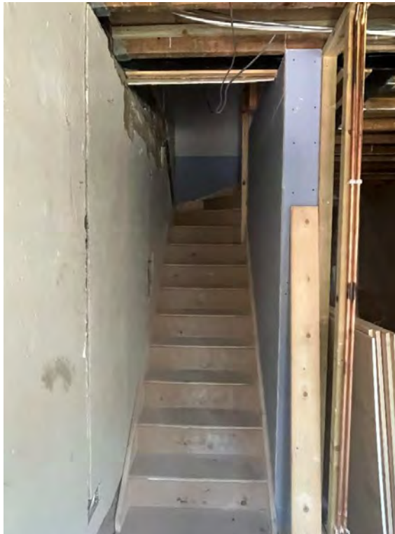
Plate 14 – New staircase installed to the centre of the building against the west wall.
