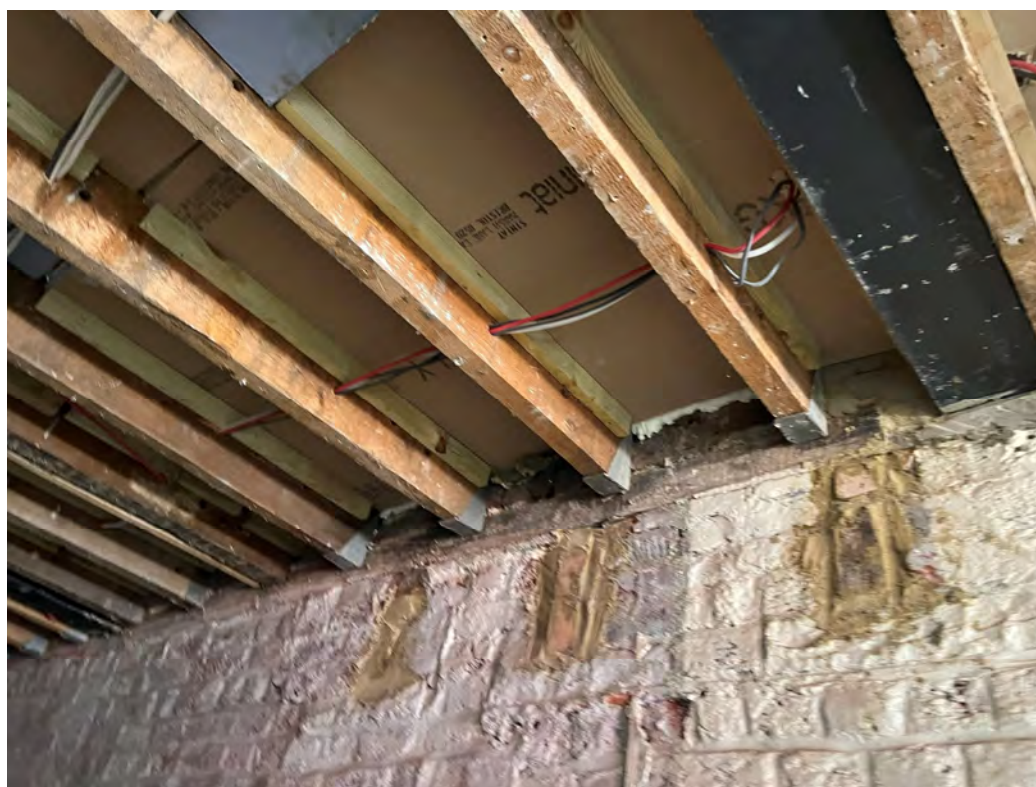
Plate 16 – Existing modern joists uncovered as part of the refurbishment works.
