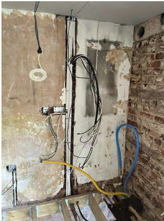
Plate 26 - New services installed to the second floor which have reused the routes of existing services to minimise disturbance to fabric.
