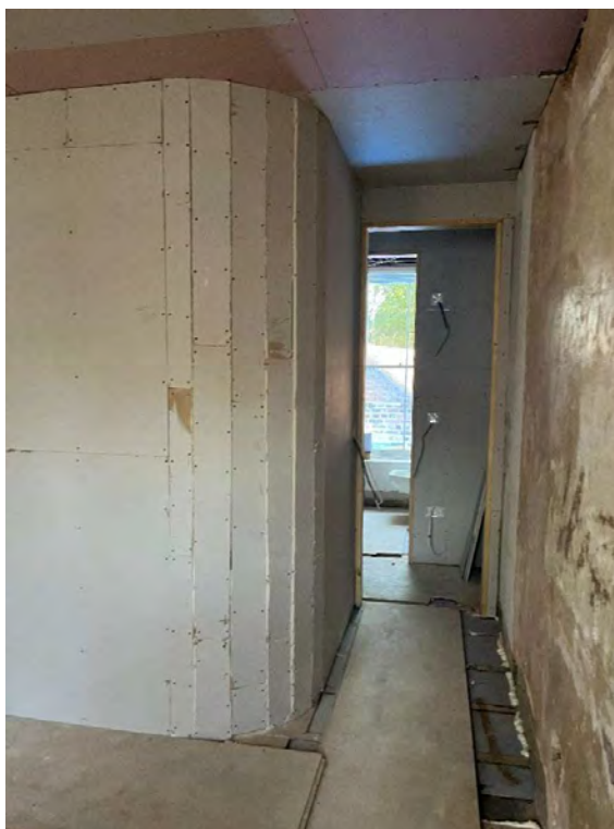
Plate 21 – View through the first floor with new stair enclosure and partition wall.
