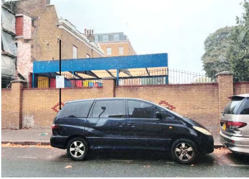
LOCATION A WITH POLE
