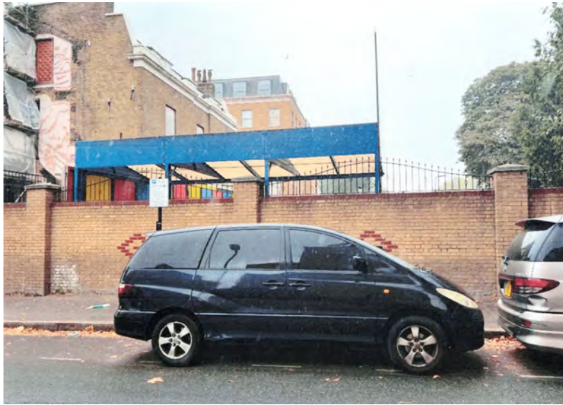
LOCATION A WITHOUT POLE
