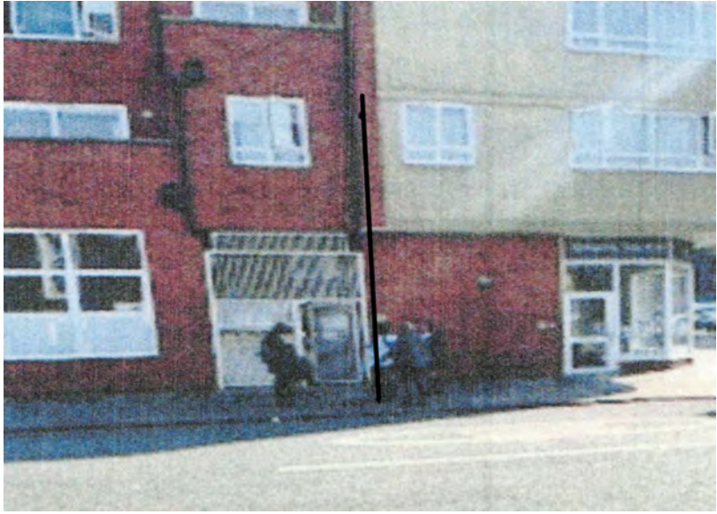
LOCATION A WITH POLE
