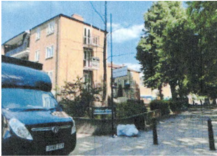
LOCATION B EXISTING
