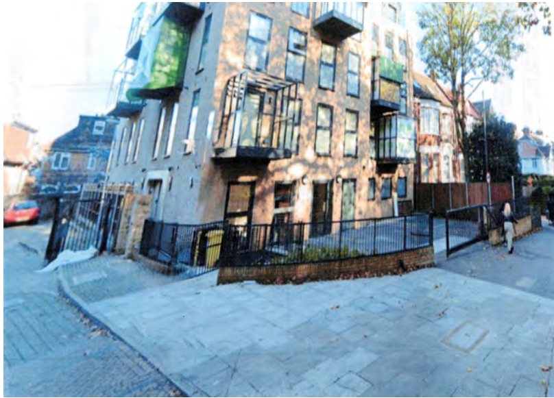
LOCATION A WITHOUT POLE
