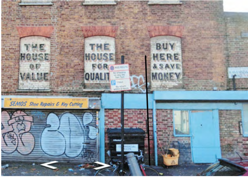
LOCATION A WITH POLE
