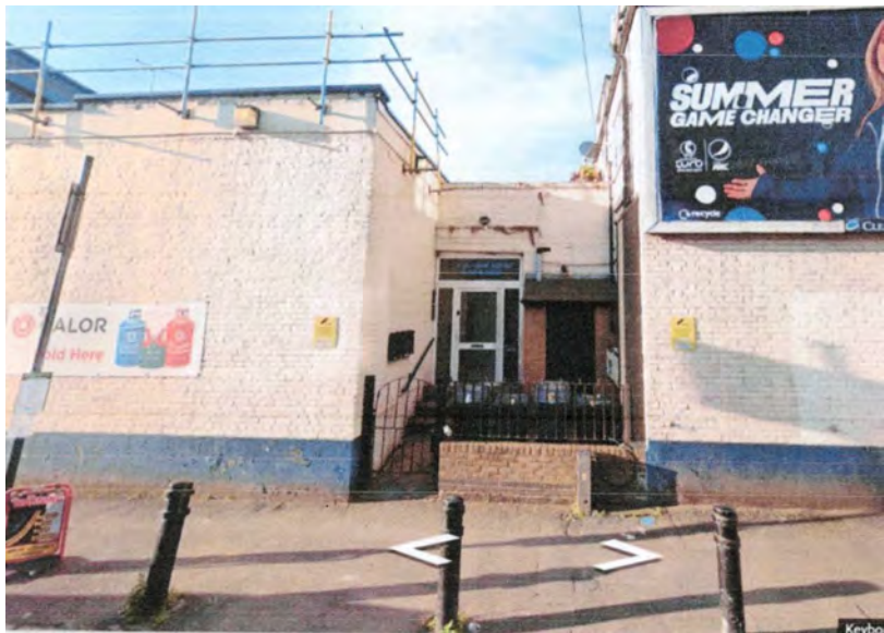
LOCATION A WITHOUT POLE
