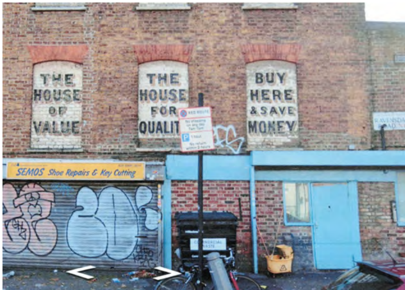
LOCATION A WITHOUT POLE
