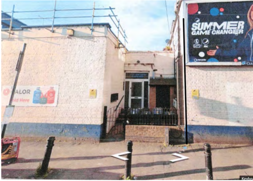
LOCATION A WITH POLE
