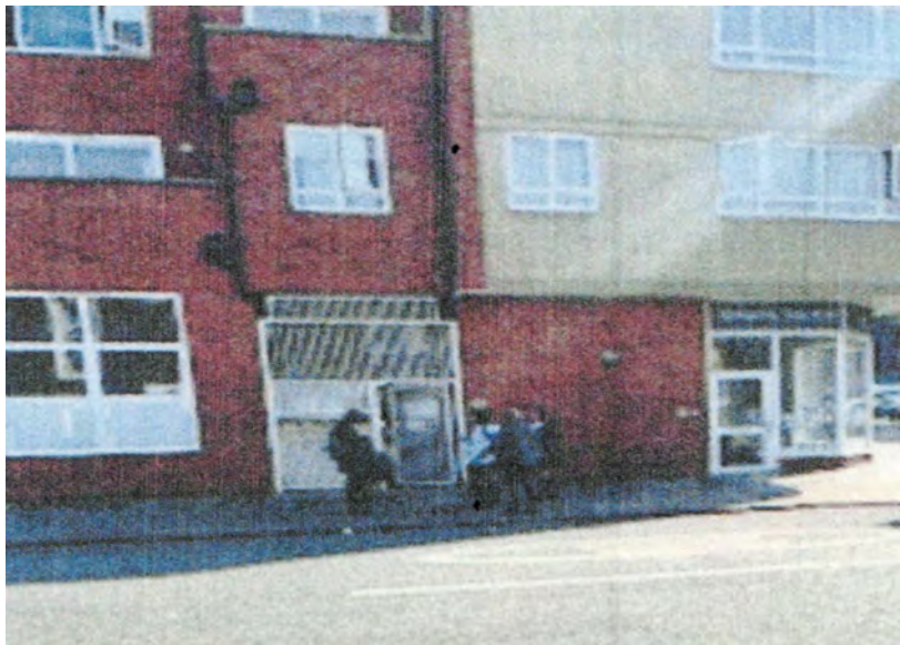
LOCATION A WITHOUT POLE
