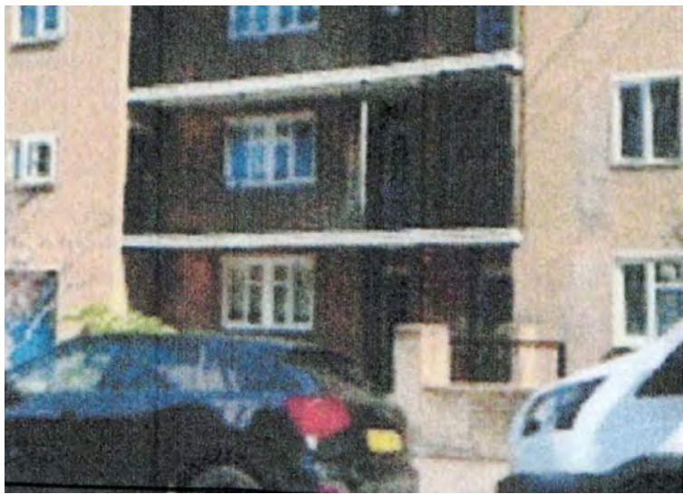
LOCATION A WITHOUT POLE
