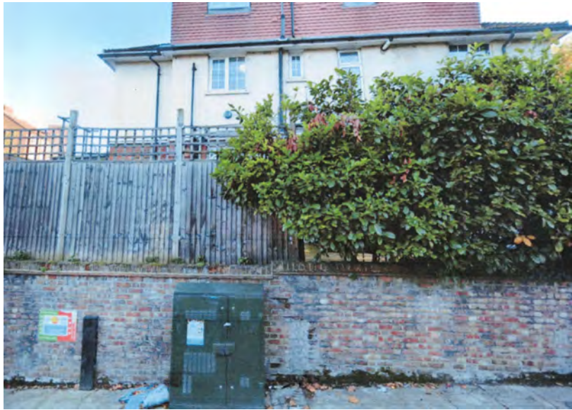
LOCATION A WITHOUT POLE
