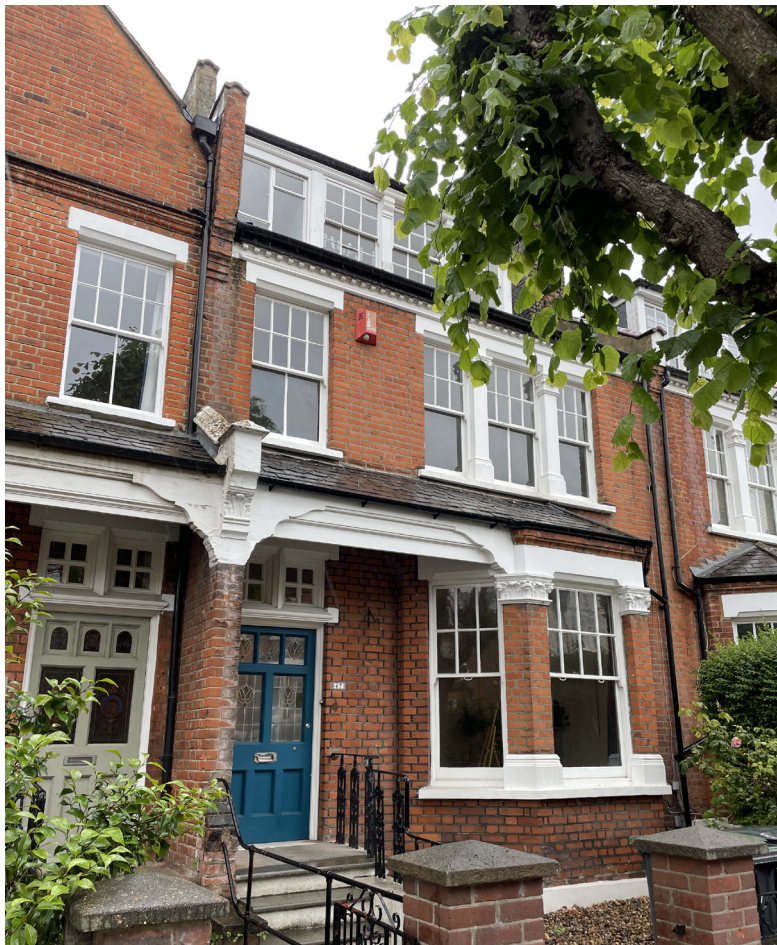
(Fig. 01) Street facing elevation of 67 Ridge Road.
