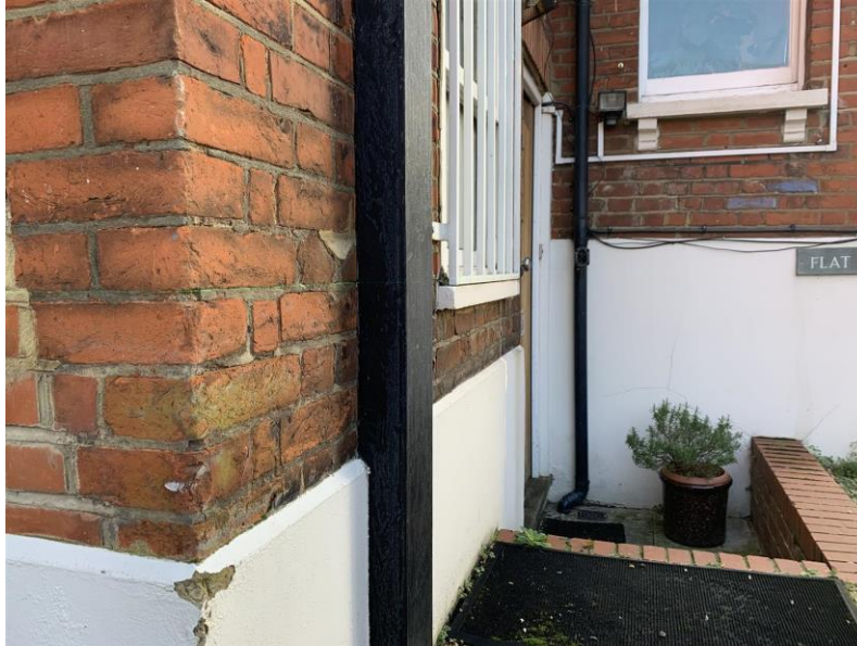
Laser line (green) shows level brickwork externally
