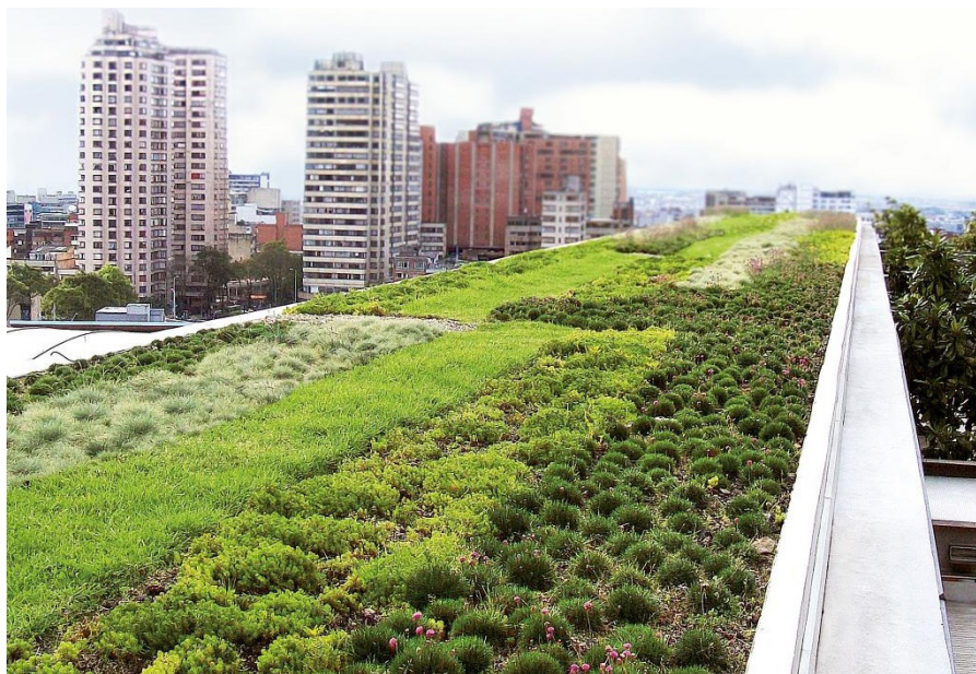
FIGURE 26 - EXTENSIVE GREEN ROOF BY ZINCO GREEN ROOF SYSTEMS
